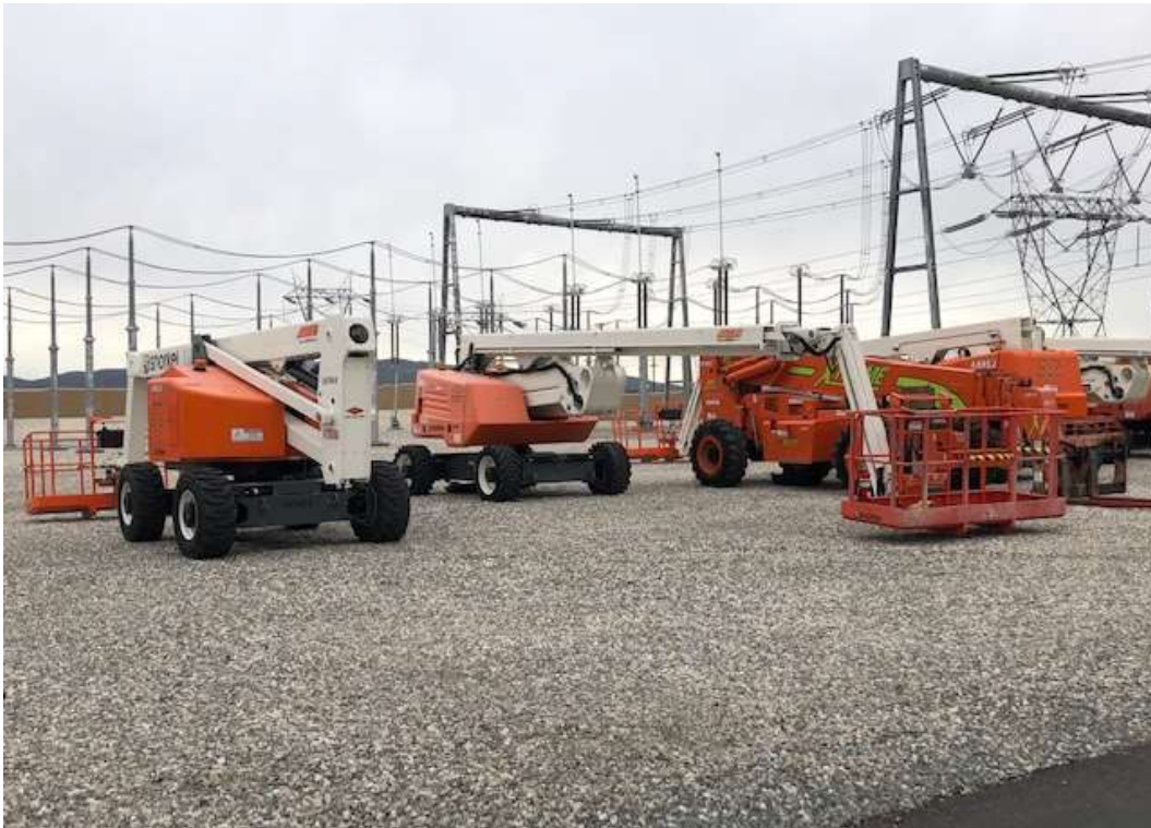
Photo 1: Work on pause at Lugo Substation (January 13, 2022).
