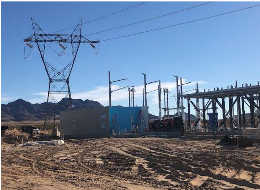
Photo 2: Progress on MEER building, Ludlow Series Capacitor (January 3, 2022).
