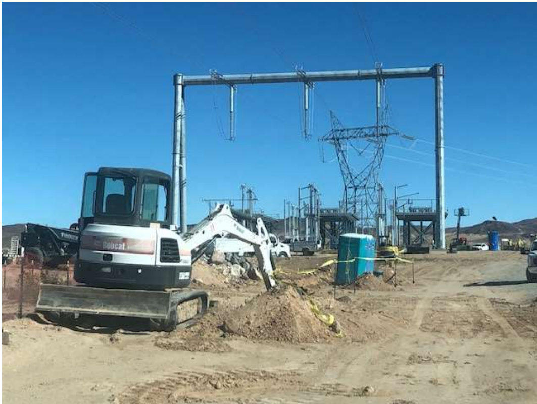
Photo 3: Trenching at Ludlow Series Capacitor (January 25, 2022).
