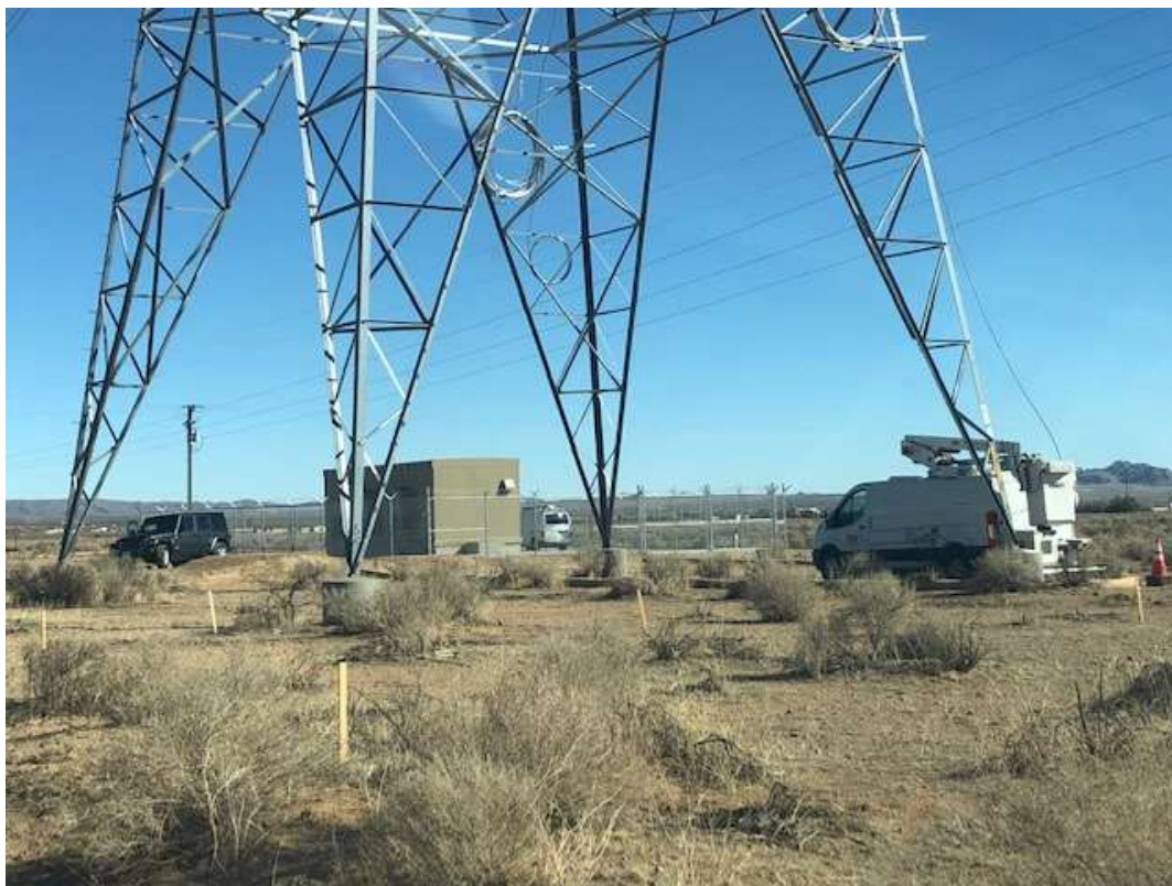
Photo 4: Completed construction along Lugo-Mohave transmission line, Barstow Repeater (January 25, 2022).
