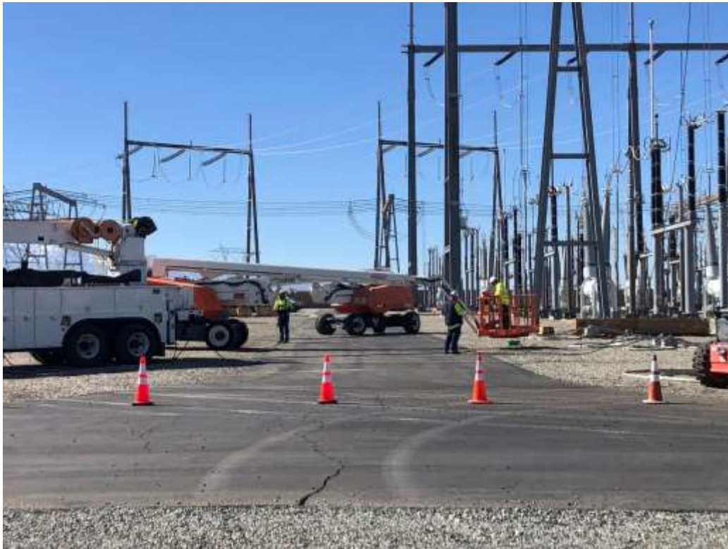
Photo 1: Construction mobilization at Lugo Substation (February 16, 2022).
