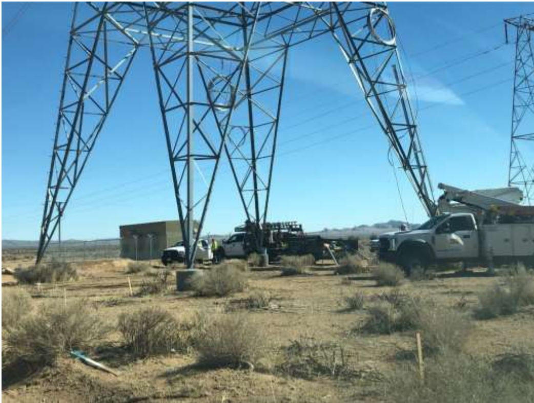
Photo 5: Completed construction at Barstow Repeater along Lugo-Mohave transmission line (February 16, 2022).
