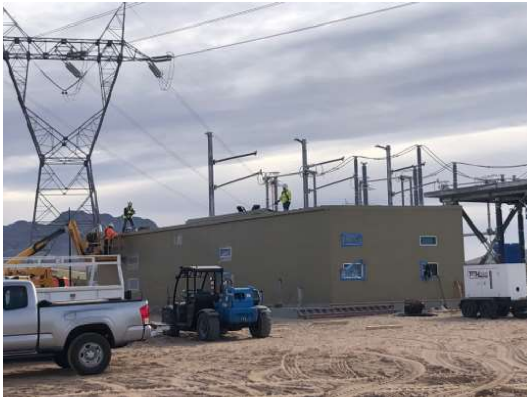
Photo 2: Progress on MEER building, Ludlow Series Capacitor (February 1, 2022).
