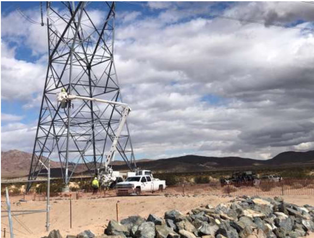
Photo 4: Wire pulling along Lugo-Mohave transmission line (February 22, 2022).
