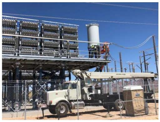
Photo 5: Capacitor installation at Ludlow Midline (April 13, 2022).
