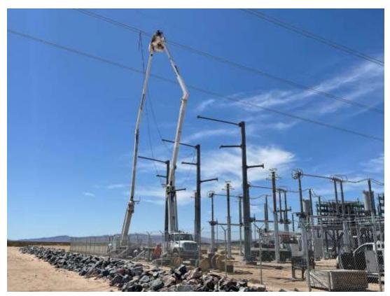
Photo 8: Wire pulling at Ludlow Midline and M69-T1 (May 5, 2022).
