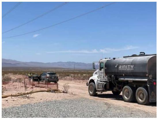
Photo 7: Dust control and escorting at Ludlow Midline (July 13, 2022).
