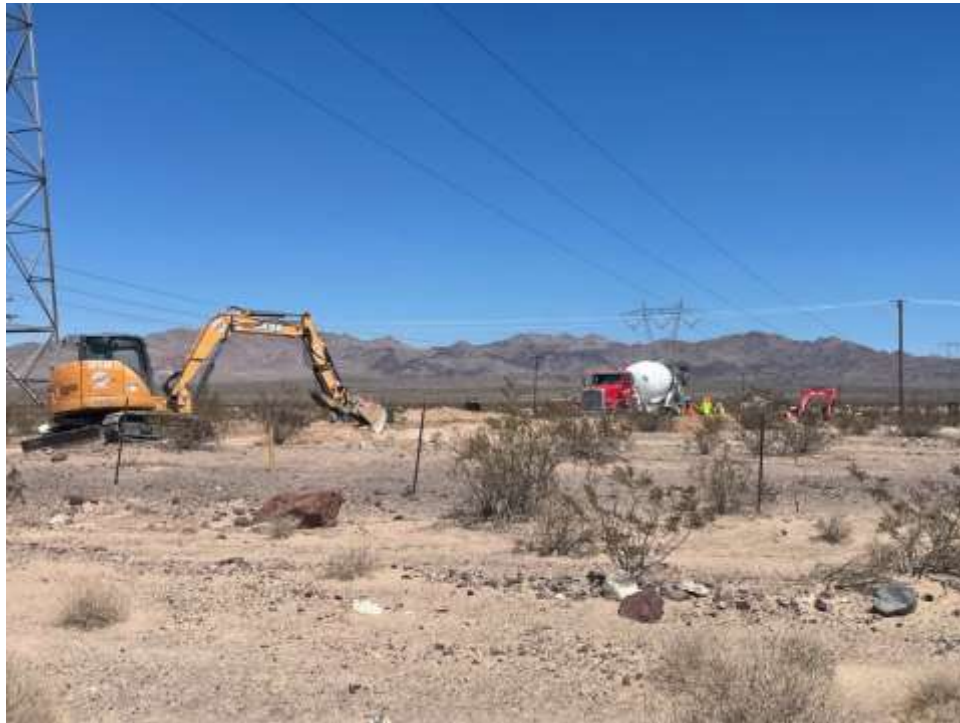
Photo 2: Conduit excavation outside SC2, Hector Way (August 30, 2022).
