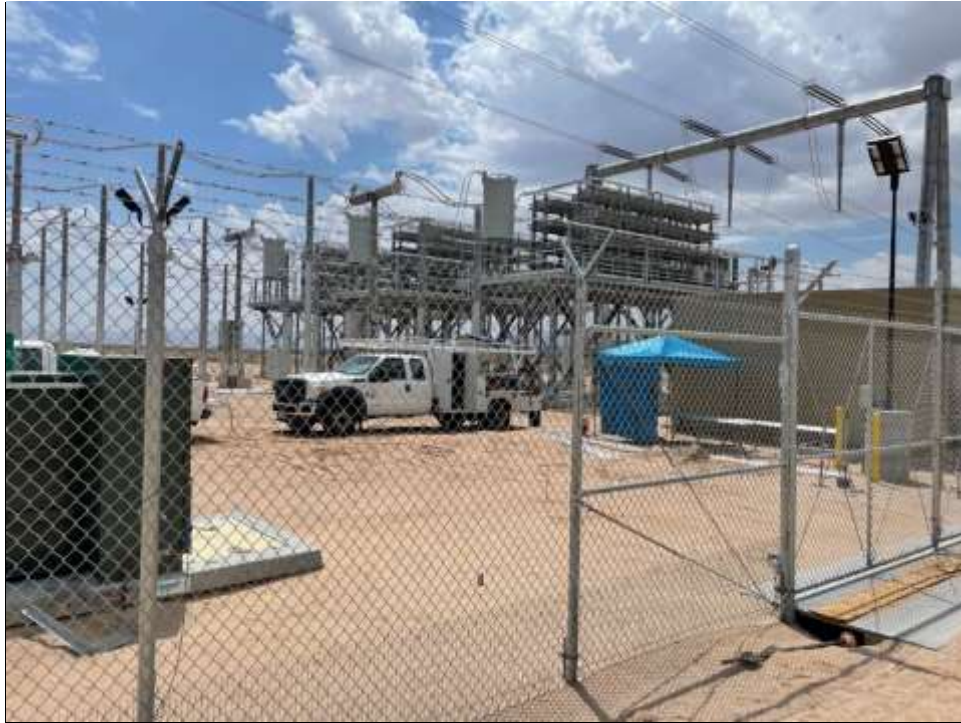
Photo 1: Decontamination/cleaning of MEER building (August 18, 2022).
