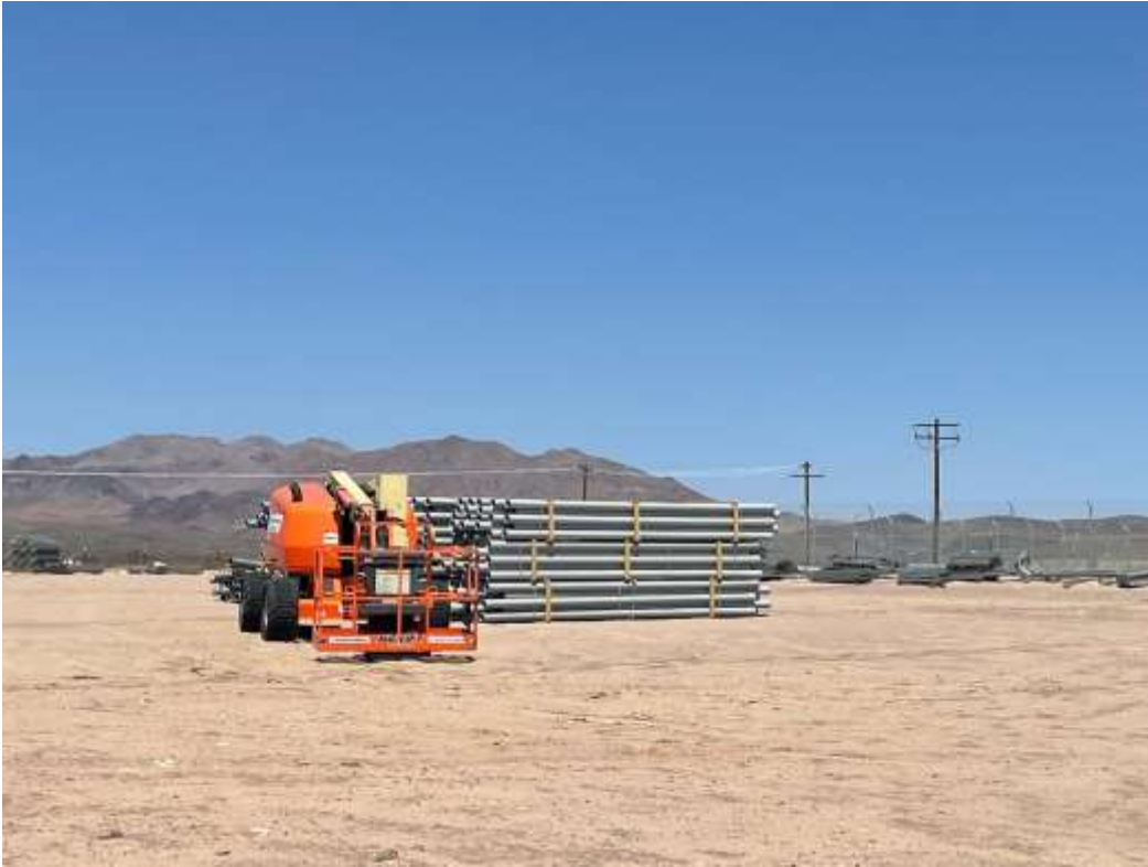
Photo 1: Staged construction materials at SC5, Ludlow Mid-line (September 7, 2022).
