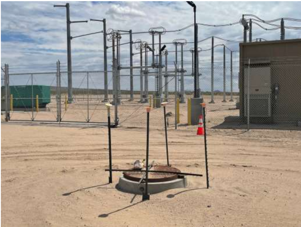
Photo 2: Completed conduit in SC5 (September 12, 2022).
