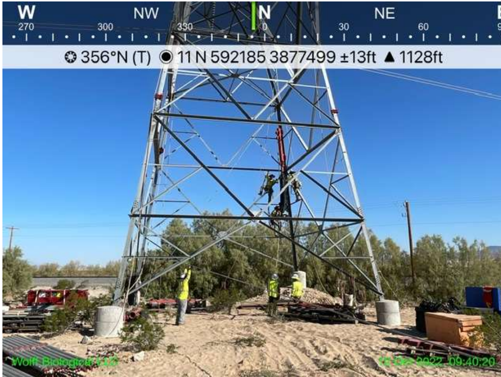
Photo 3: Ampjack crew at M97-T1 (October 12, 2022; photo by Beth Wolff, EPG).
