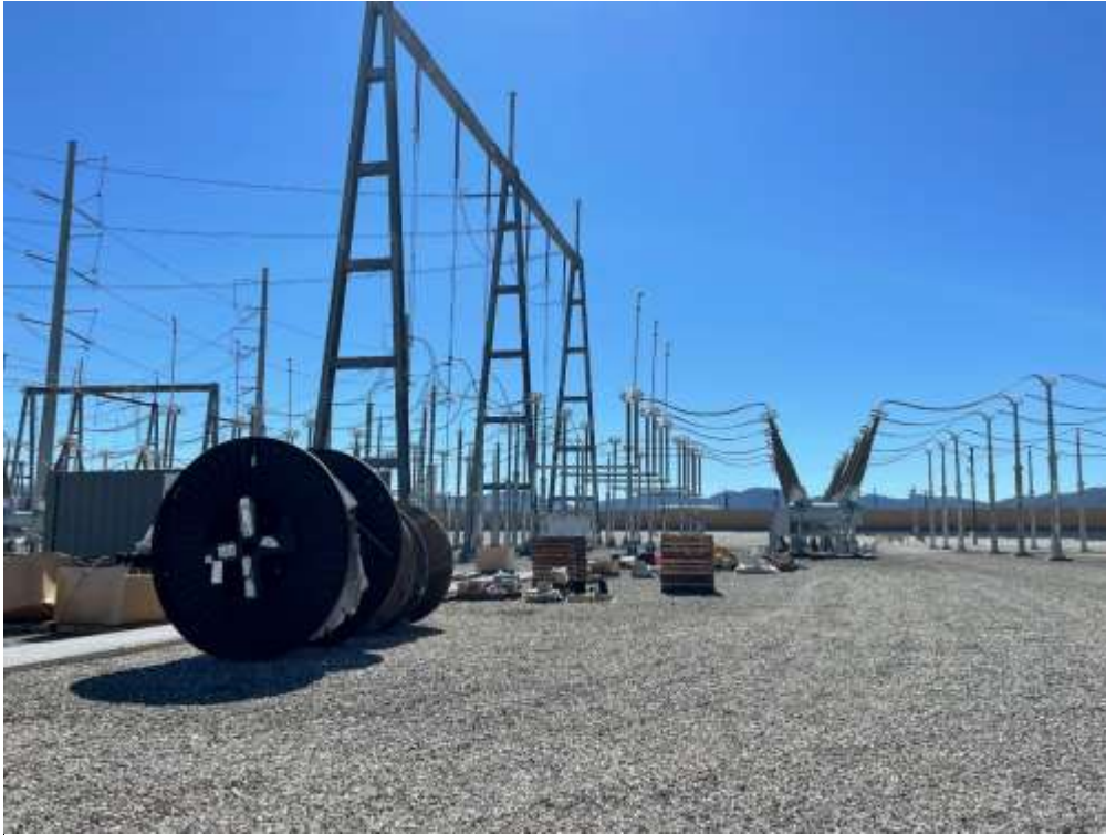
Photo 1: Staged construction materials at SC4, Lugo Substation (October 18, 2022).
