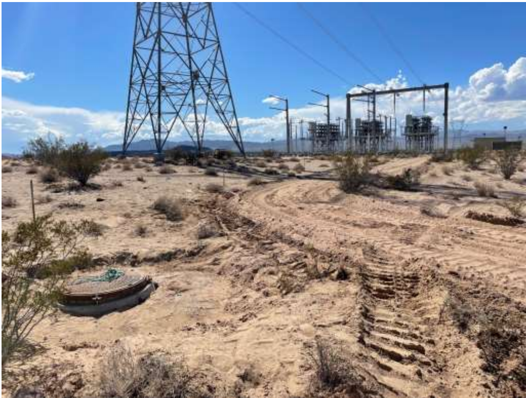
Photo 4: Site of previous wire-stringing outside SC5 (October 11, 2022).
