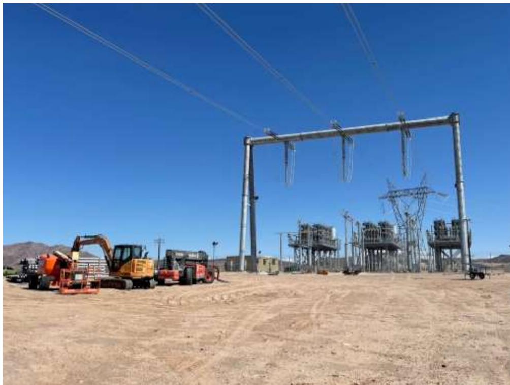
Photo 2: Staged equipment at SC5, Ludlow mid-line (October 11, 2022).
