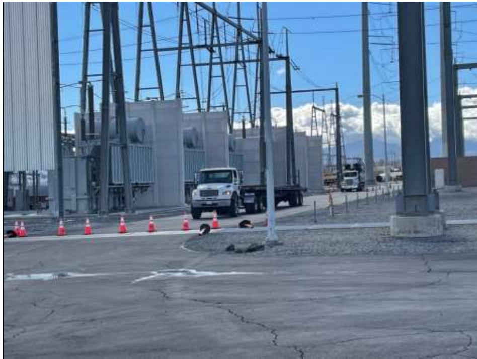
Photo 1: Mobilization of construction materials at SC4, Lugo Substation (November 9, 2022).
