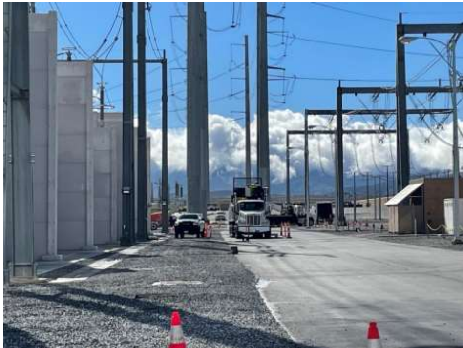
Photo 2: Mobilization of construction materials at SC4, Lugo Substation (November 9, 2022).
