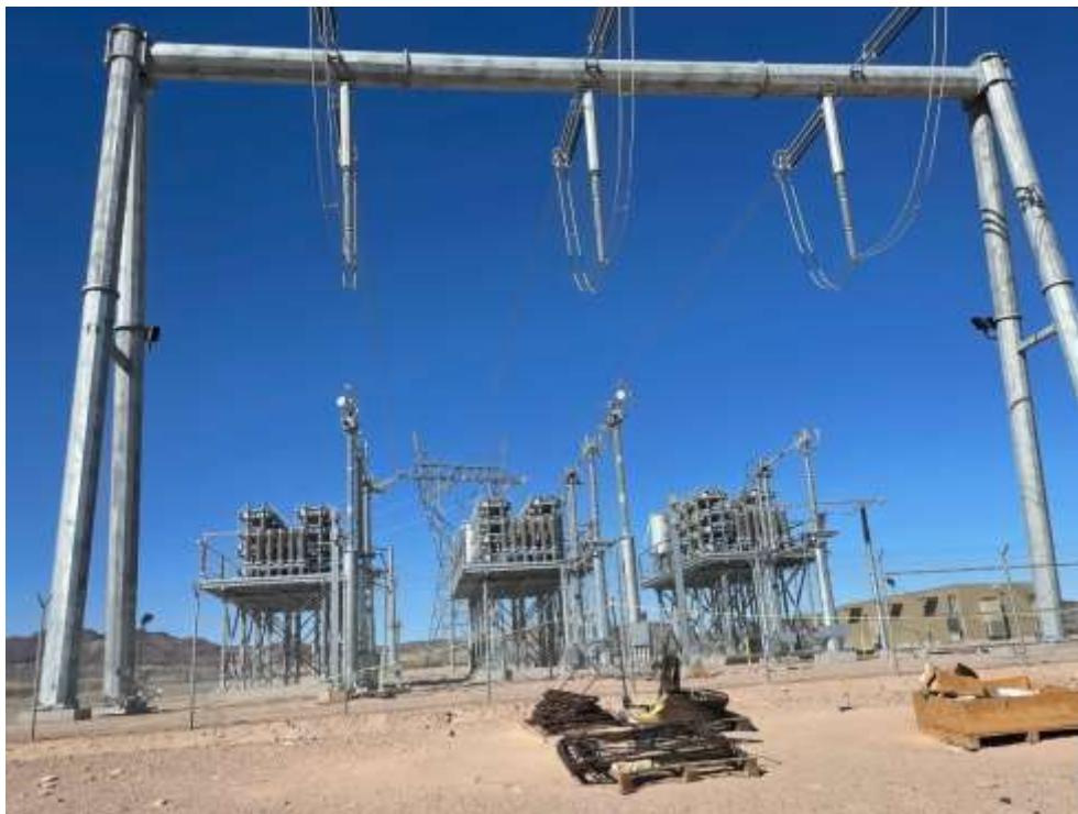
Photo 4: Staged equipment at SC5, Ludlow mid-line (November 14, 2022).
