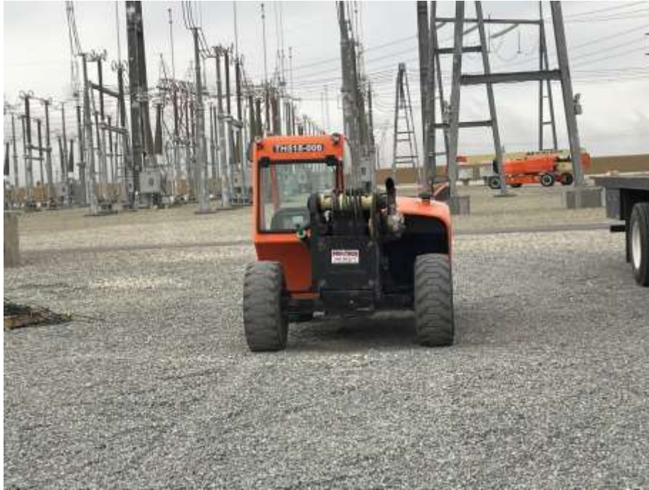
Photo 1: Wire stringing equipment at SC4, Lugo Substation (December 1, 2022).
