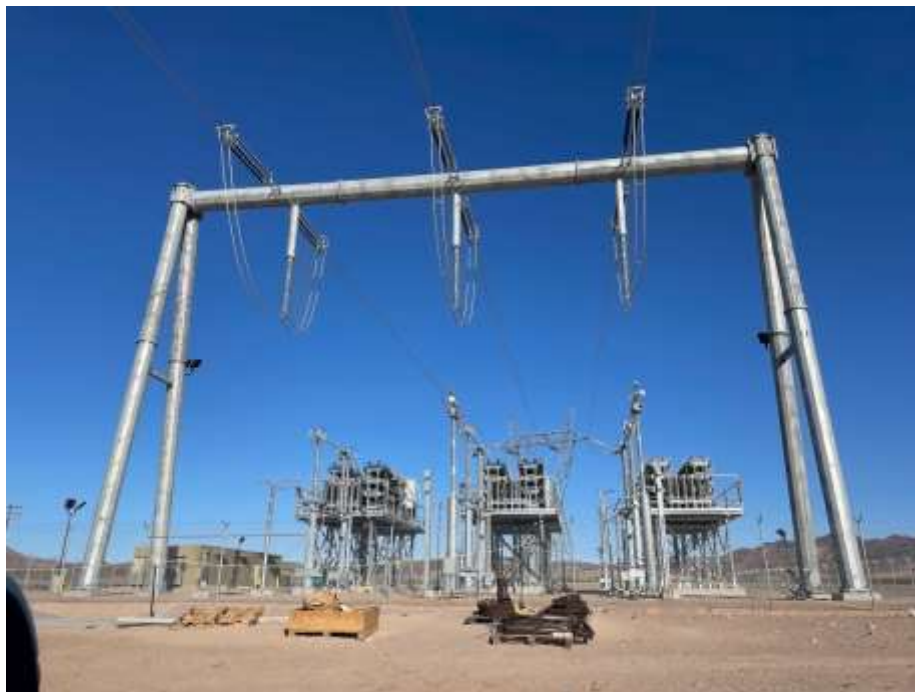
Photo 4: Staged equipment at SC5, Ludlow mid-line (December 14, 2022).
