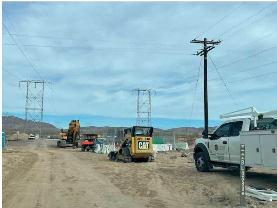
Photo 2: Trenching and foundation pouring outside SC5 (January 11, 2023).
