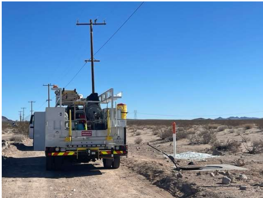
Photo 4: Wire stringing outside SC5 (January 25, 2023).
