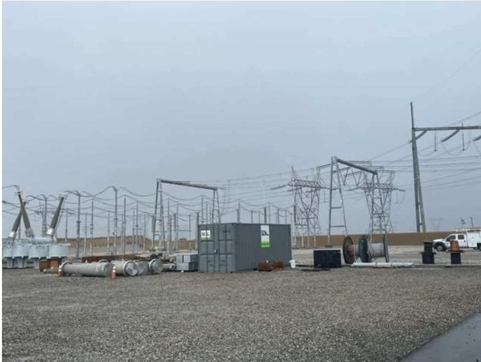
Photo 1: Staging materials at SC4, Lugo Substation (January 5, 2023).
