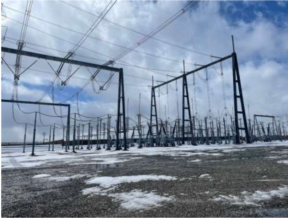
Photo 1: Paused construction in snow at SC4, Lugo Substation (February 27, 2023).
