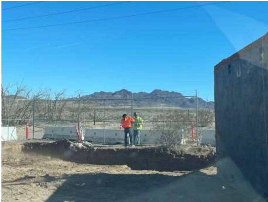
Photo 2: Trenching and foundation pouring outside SC5, Ludlow Midline (February 1, 2023).
