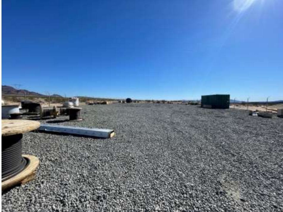
Photo 3: Laydown yard for material staging at SC5, Ludlow Midline (February 1, 2023).
