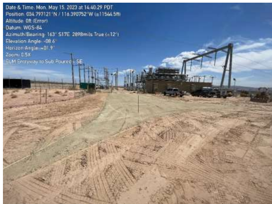
Photo 4: Entryway into Ludlow capacitor poured and complete to final grade (May 15, 2023).
