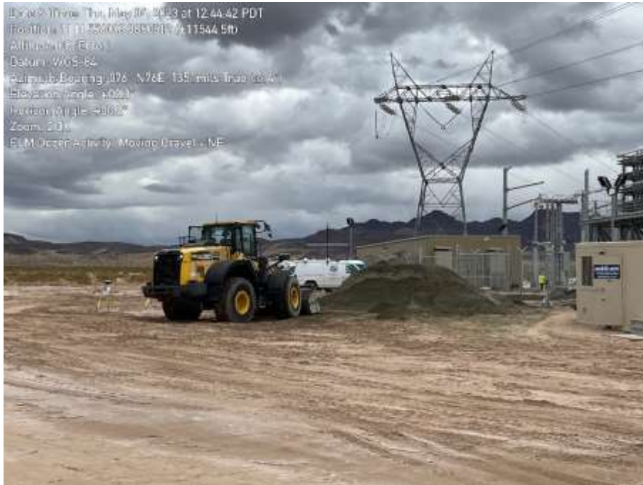
Photo 1: Delivery and distribution of gravel material, SC5 (May 4, 2023).
