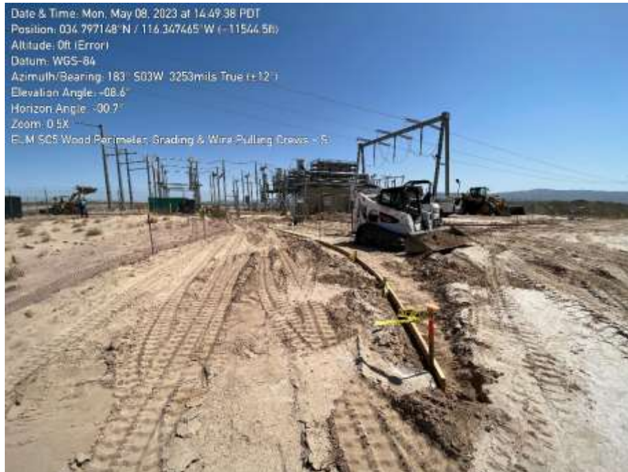
Photo 3: Bringing site to final grade, SC5 (May 8, 2023).
