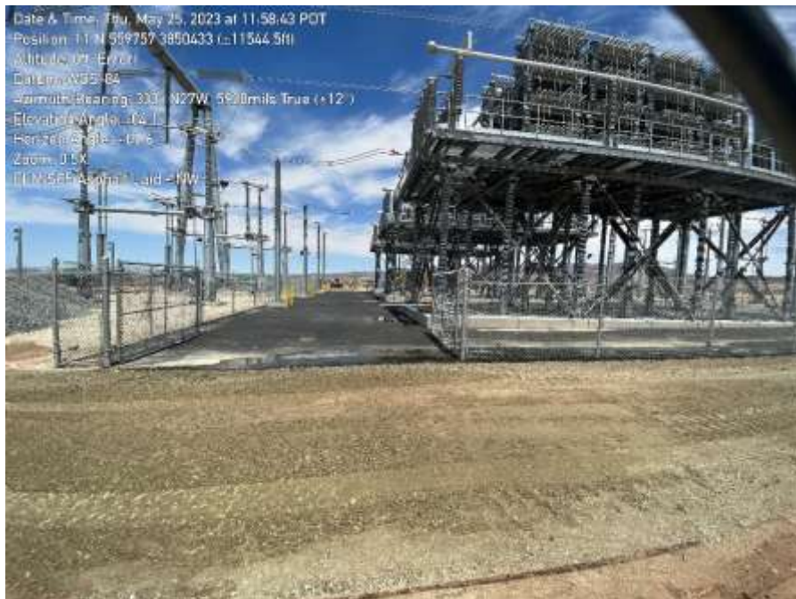
Photo 2: Asphalt poured surrounding the Ludlow capacitor, SC5 (May 25, 2023).
