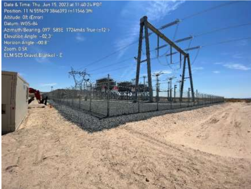
Photo 3: SC5 brought to final grade. Photograph from June 15th.
