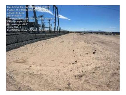
**Photo 3**: Post-Hurricane Hilary conditions at SC5. No erosion or storm damage observed along the capacitor's southern-border drainage/V-ditch (pictured, facing SW).
