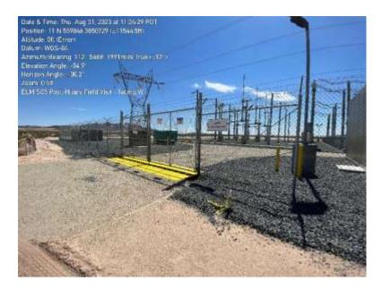
**Photo 2**: Post-Hurricane Hilary conditions at SC5. No erosion or storm damage observed at/surrounding one of the capacitor's entrance gate (facing west).
