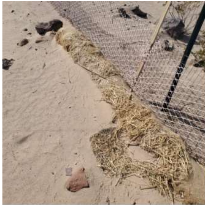
Photo 1: Perimeter wattle deterioration/damage at SC5. Photo courtesy of site SWPPP QSP.
