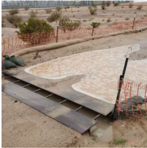
Photo 3: Ponding water at SC2 entrance, after documented rain events occurring on February 1 st , and February 4 th . Post-rain event on-site inspections were conducted by the project QSP in accordance with the project's SWPPP storm reporting requirements. Photo courtesy of site QSP, SWPPP inspection conducted on February 6 th , 2024.
