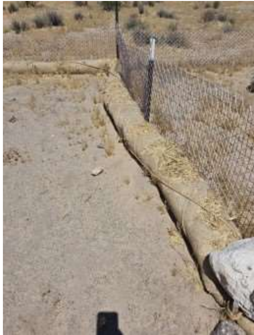
Photo 5: Damaged perimeter wattle at SC5, with evident large holes and animal damage. Photo courtesy of site QSP, SWPPP inspection conducted on June 25, 2024.
