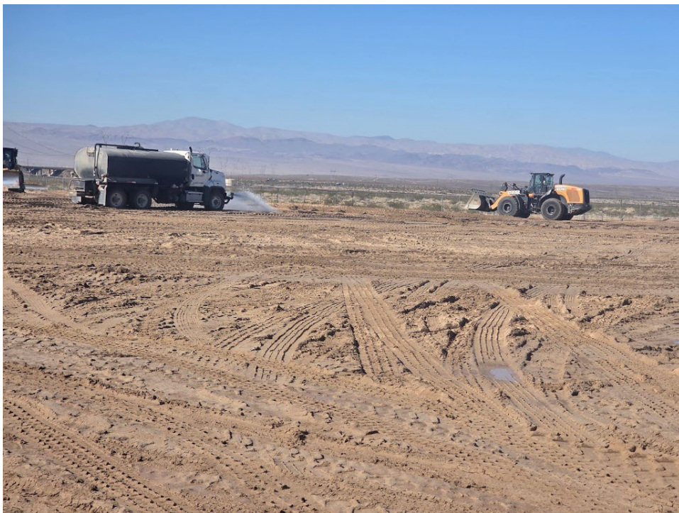
Photo 2. Construction of the Ludlow Yard (October 1, 2025).
