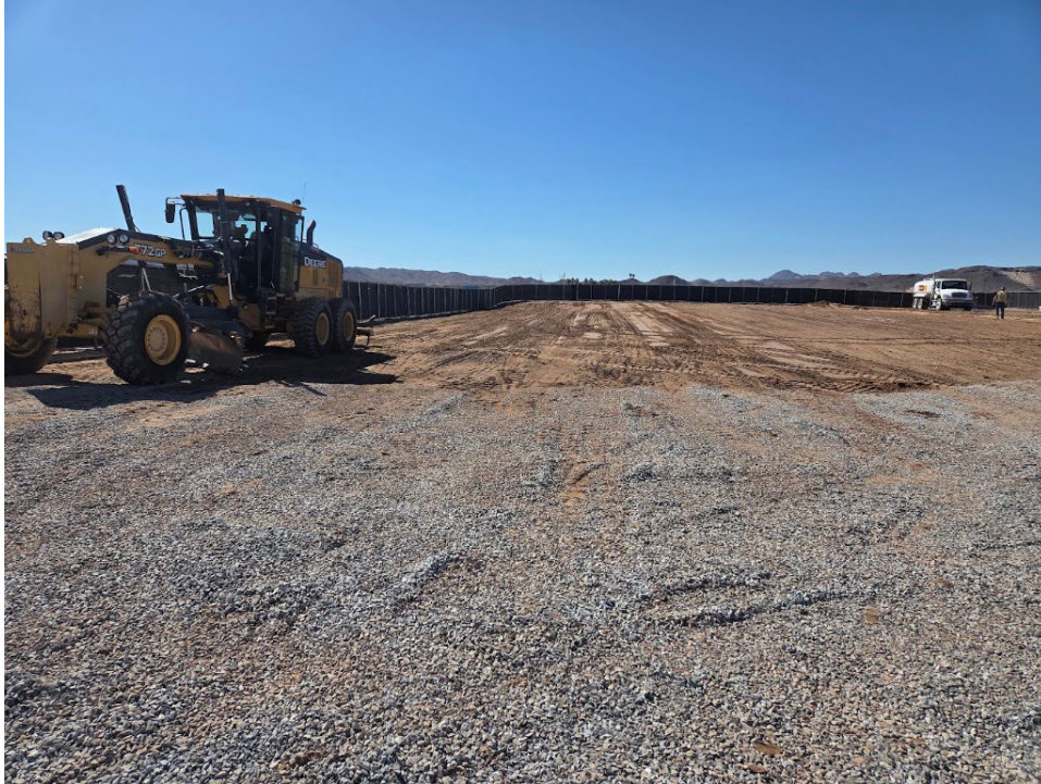
Photo 1. Construction of the Crucero Road Yard (September 24, 2025).
