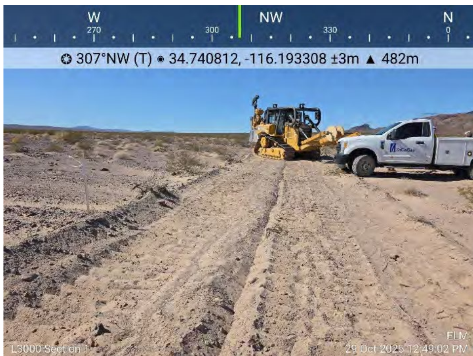
Photo 6. L3000 Section 1 V-ditch Trencher (October 29, 2025) (Photo Provided by SoCalGas)
