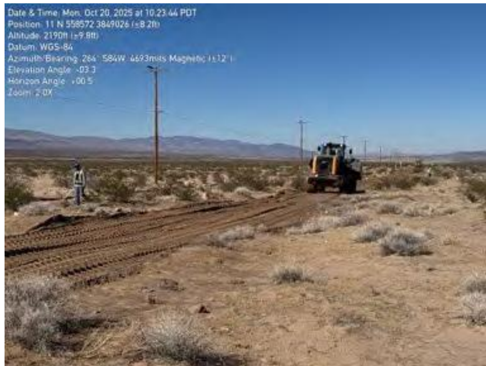
Photo 3. L235 Section 20 Restoration Grading (October 20, 2025) (Photo Provided by SoCalGas)
