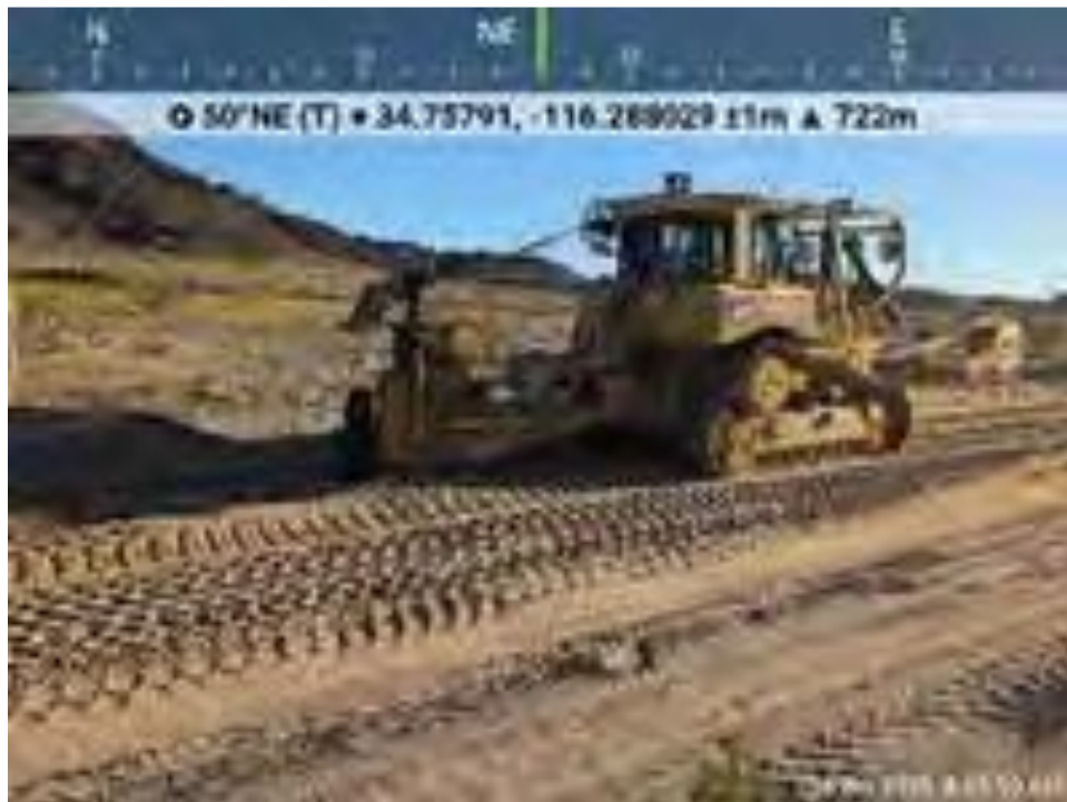
Photo 5. Ripping at L235 Section 17A (Photo provided by So Cal Gas)
