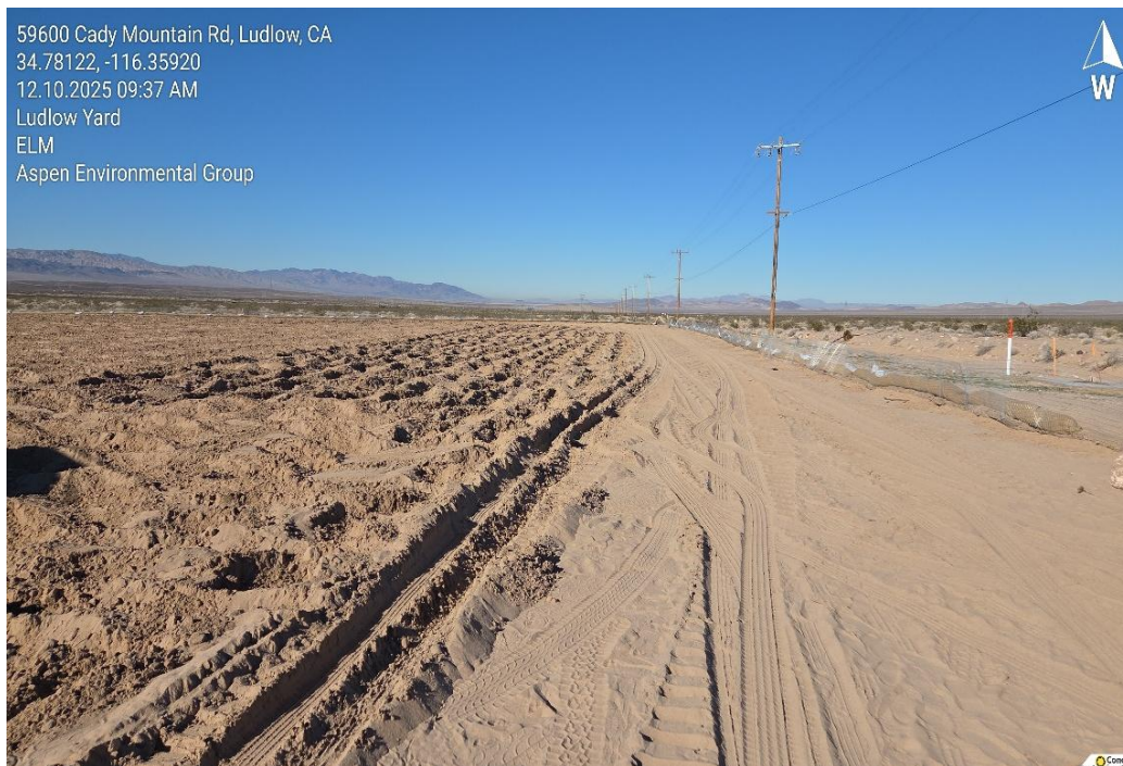
Photo 2. Ludlow Yard decompaction and fence removal (December 4, 2025).
