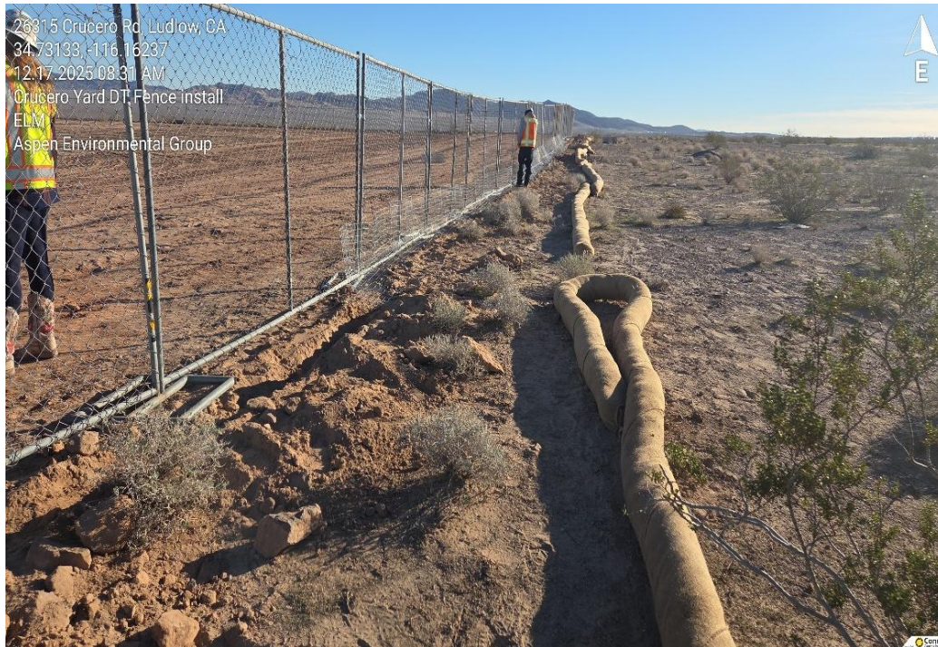
Photo 1. Crucero Yard Security and Desert Tortoise Fence Installation (December 17, 2025).
