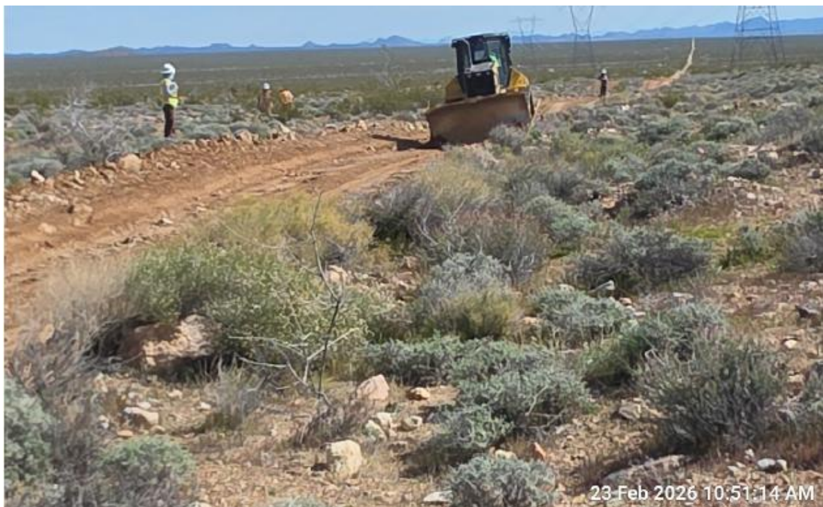
Photo 4. L235 Section 2 Site Restoration (February 23, 2026) (Photo courtesy of SoCalGas)
