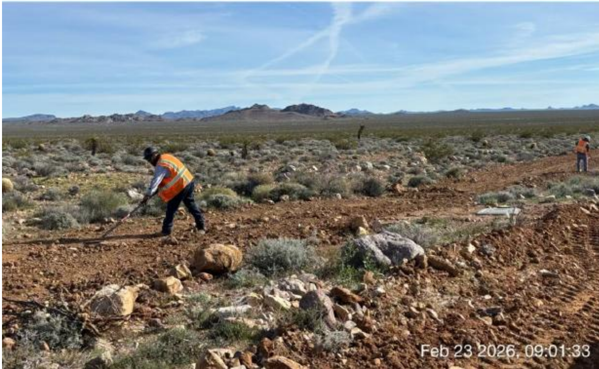
Photo 3. L235 Section 1 Site Restoration (February 23, 2026) (Photo courtesy of SoCalGas)
