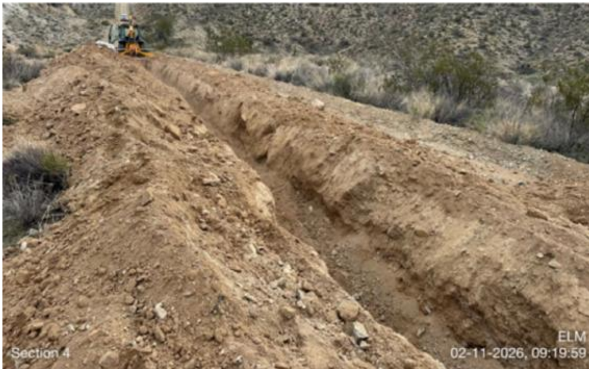
Photo 2. L235 Section 4 Wire Installation (February 10, 2026) (Photo courtesy of SoCalGas)
