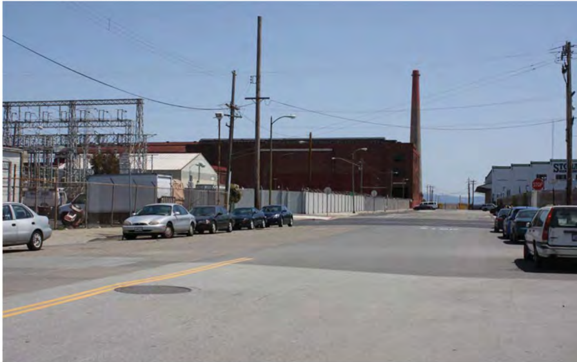
3. 23rd Street at 3rd Street looking northeast
