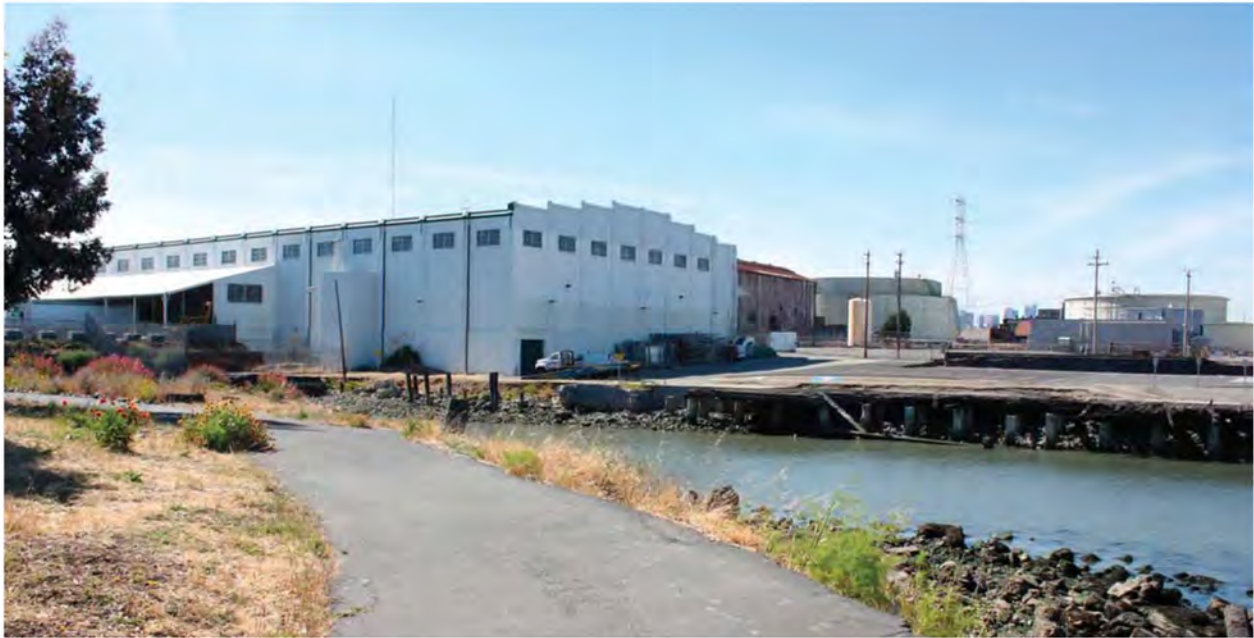
7. Warm Water Cove Park looking northwest
