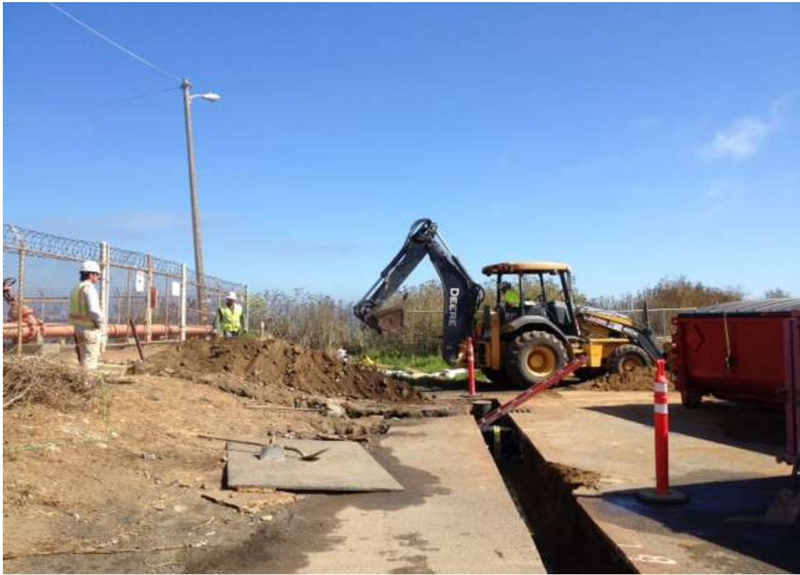
Figure 3 – Water line work on 23 rd Street. View east, October 9, 2014.
