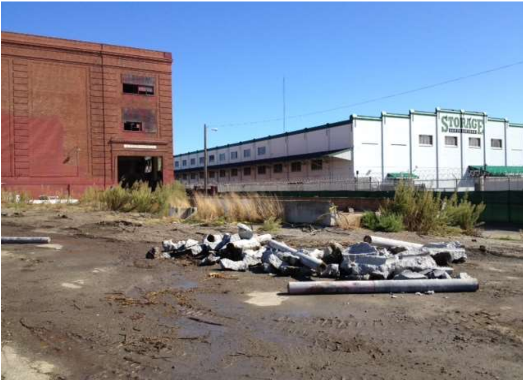
Figure 1 – Demolition and debris clean-up at Potrero Switchyard. View southeast, October 9, 2014.
