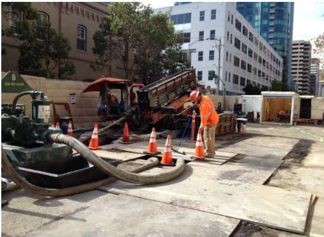
Figure 2 – HDD set-up at Bore #2 on Spear Street. View west, October 9, 2014.
