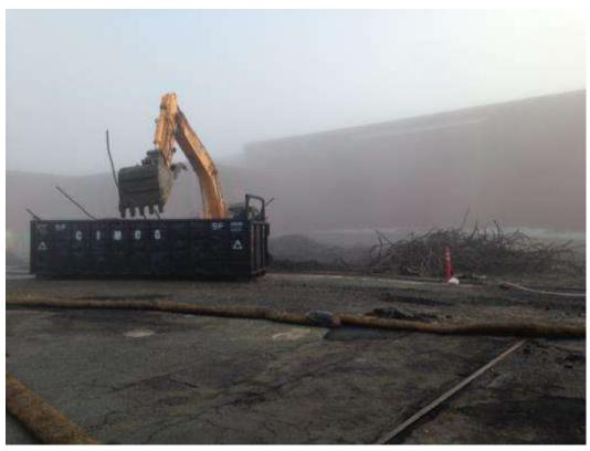
Figure 1 – Loading rebar to be hauled off and recycled at Potrero Switchyard. View northeast, December 22, 2014. Photo courtesy of PG&E.
