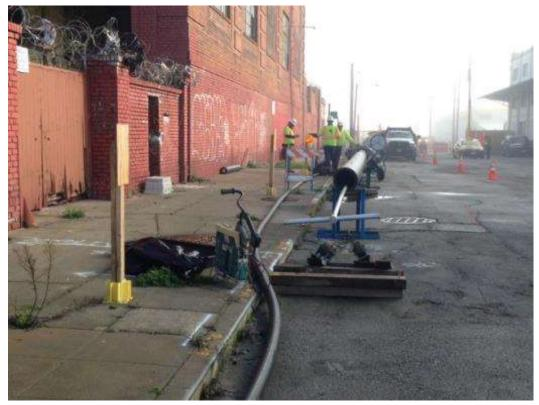
Figure 3 – HDPE fusing at HDD South along 23<sup>rd</sup> Street. View east, December 22, 2014. Photo courtesy of PG&E.
