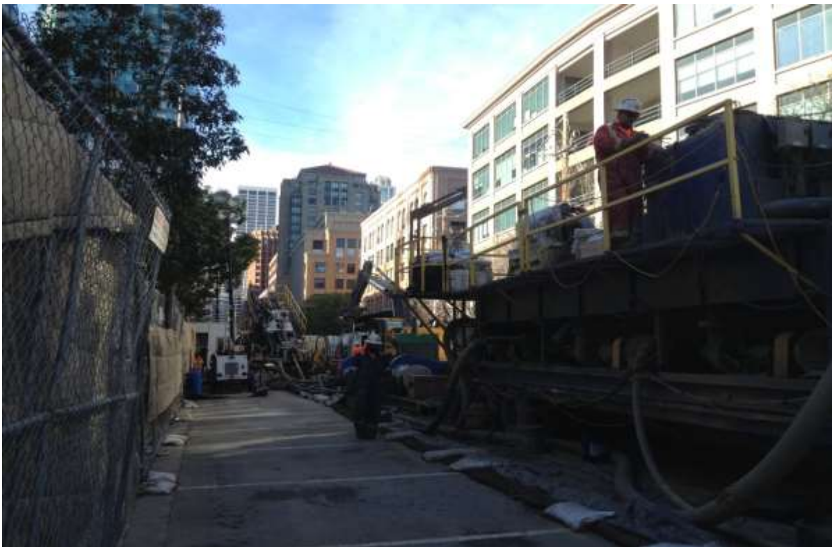
Figure 2 – HDD Company drilling at HDD North. View west, February 12, 2015.
