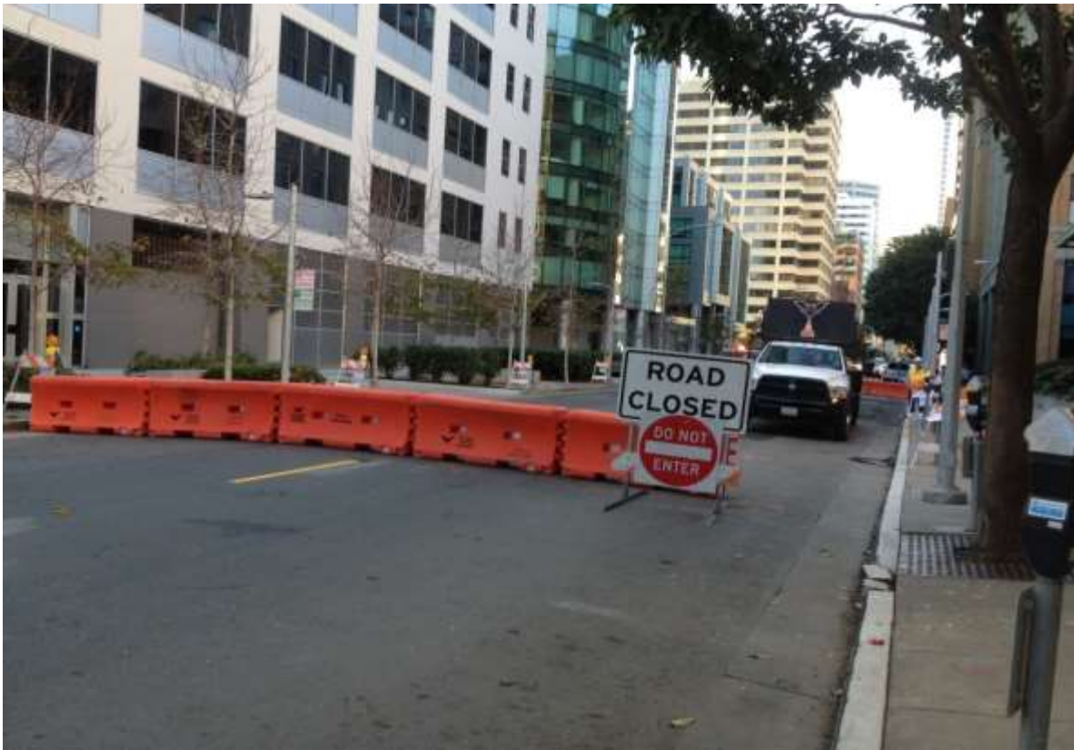
Figure 3 – Traffic controls being set-up on Spear Street. View west, February 12, 2015.
