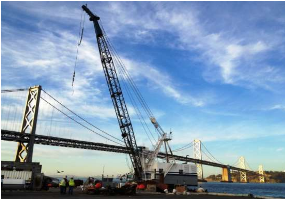
Figure 2 – Vortex set-up at HDD North – Pier 30/32. View north, February 26, 2015.
