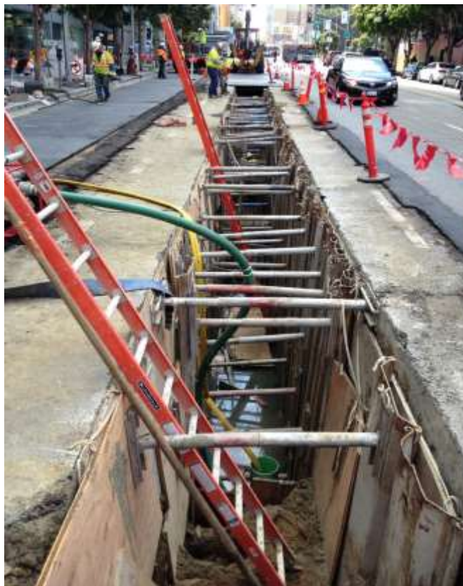
Figure 2 – Underground duct bank work on Folsom Street. View south, April 1, 2015.
