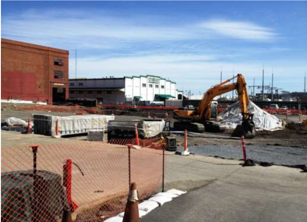
Figure 1 – Excavating at Potrero Switchyard, view southeast, April 1, 2015.
