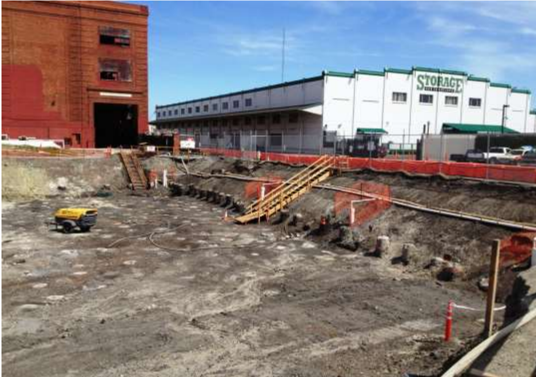
Figure 1 – Drill displacement columns (DDCs) exposed at Potrero Switchyard. View southeast, April 28, 2015.
