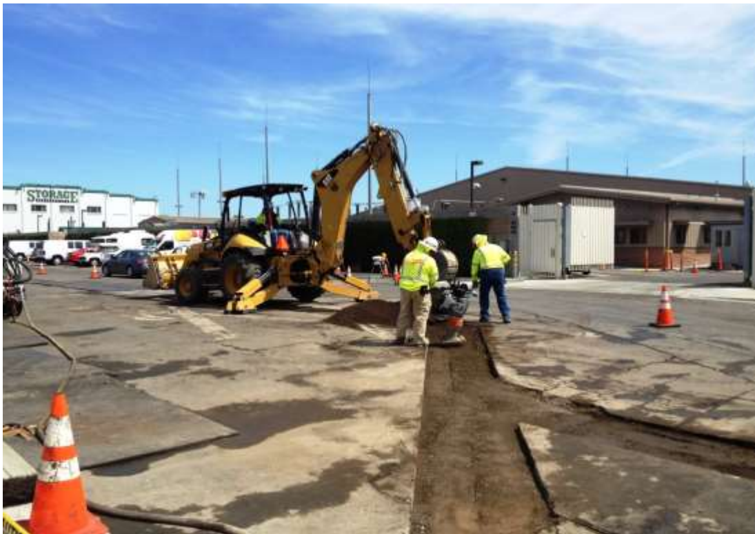
Figure 4 – Backfilling waterline trench on 23 rd Street. View southeast, April 28, 2015.
