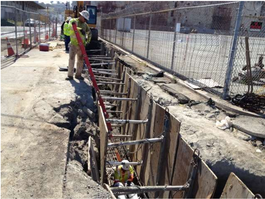
Figure 3 – Excavating duct bank trench on 23 rd Street. View west, June 4, 2015.
