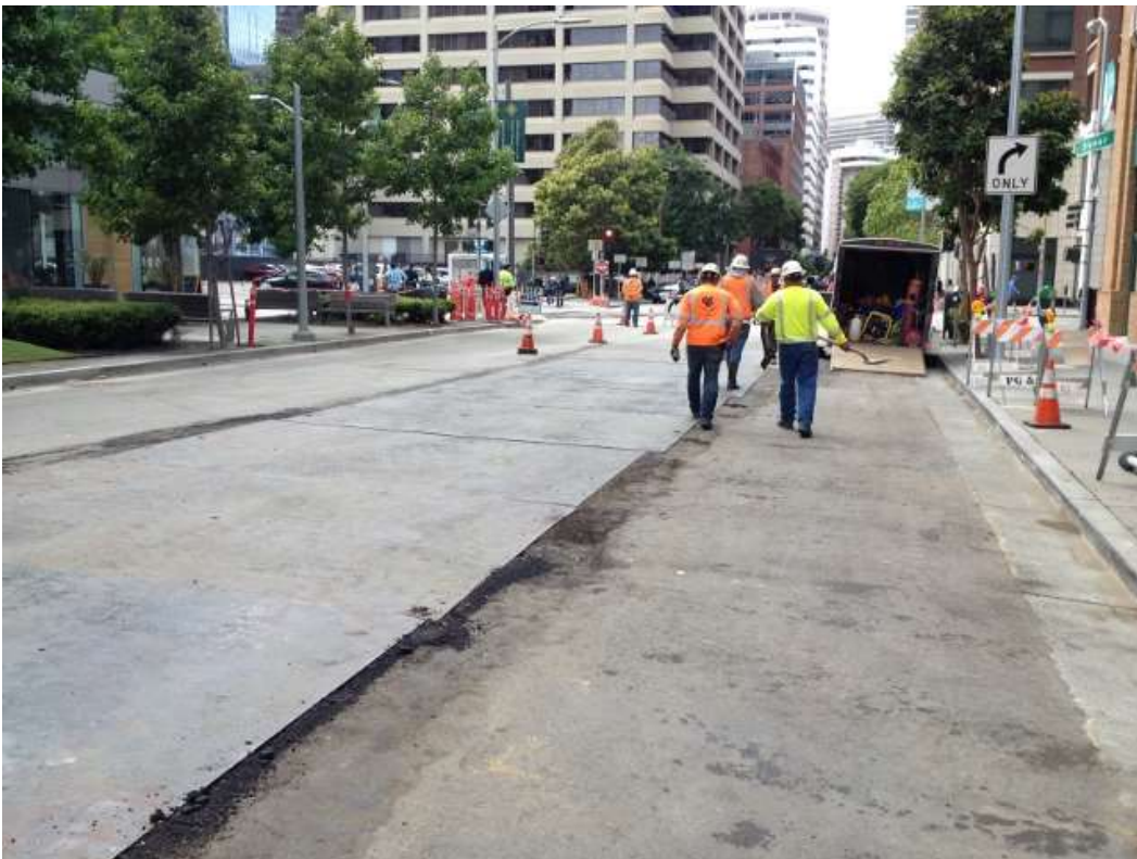
Figure 2 – Duct bank work on Spear Street. View west, July 10, 2015.
