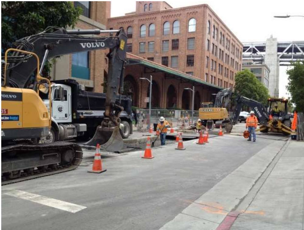
Figure 3 – Removing pavement on Spear Street. View northeast, August 21, 2015.
