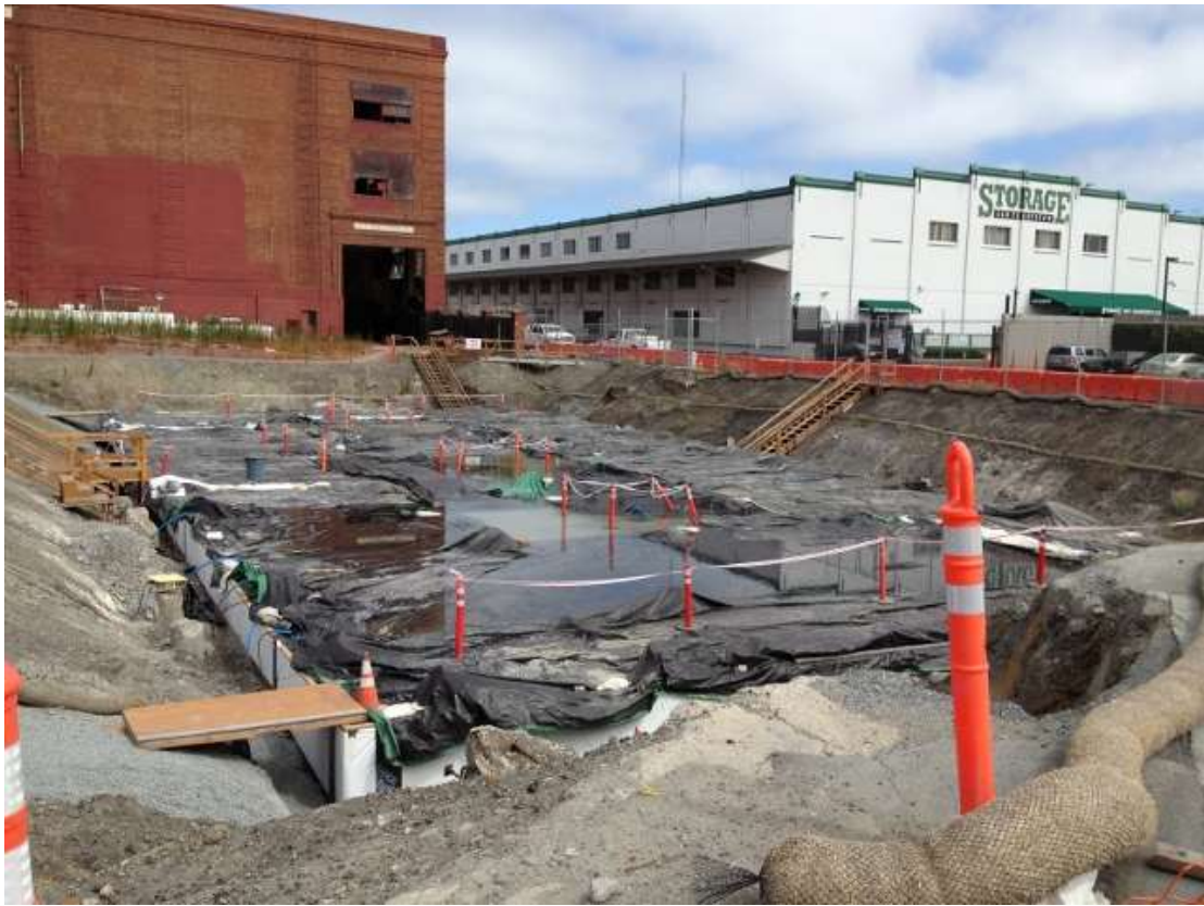
Figure 5 – Potrero Switchyard building foundation concrete curing. View southeast, August 21, 2015.
