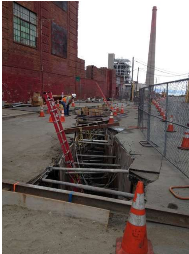
Figure 4 – Excavated and poured concrete on 23 rd Street. View east, September 14, 2015.
