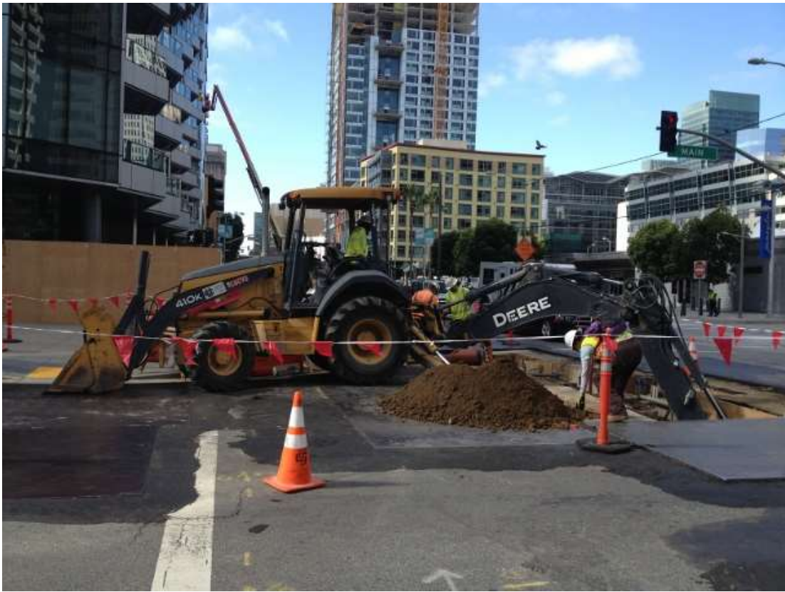
Figure 3 – Excavating trench on Folsom Street at Main Street. View southwest, October 6, 2015.
