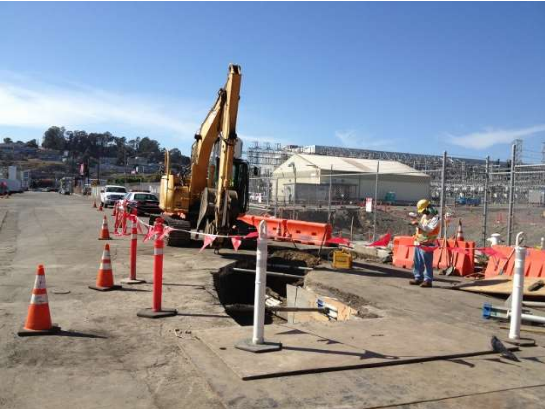
Figure 4 – Excavating trench on 23 rd Street. View west, October 6, 2015.
