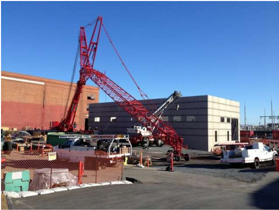
Figure 5 – Demobilizing crane at Potrero Switchyard. View southeast, November 3, 2015.
