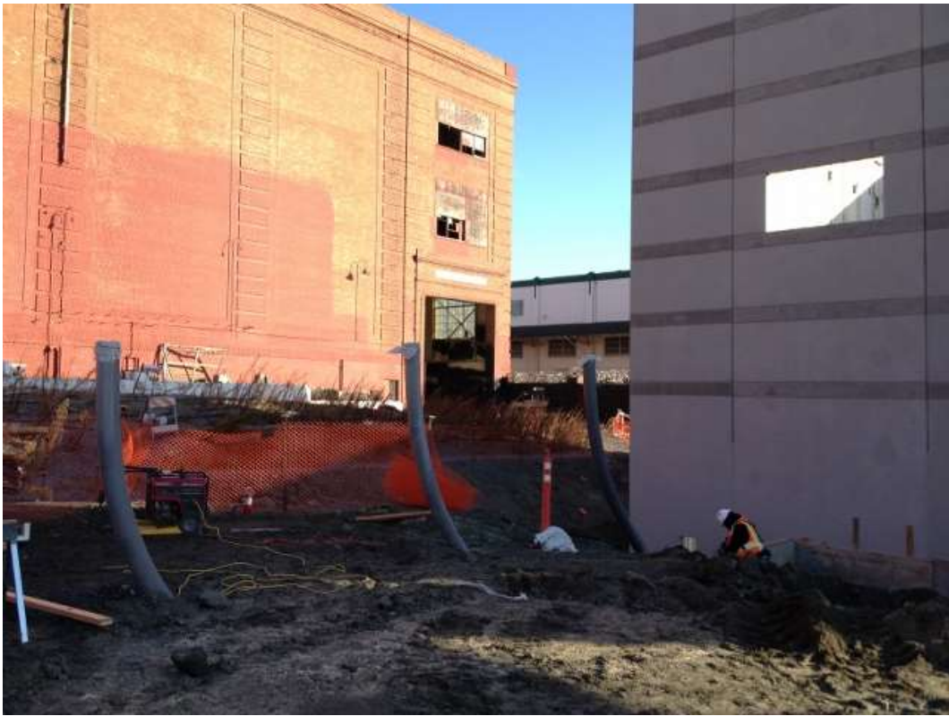
Figure 5 – Potrero Switchyard work. View southeast, November 24, 2015.
