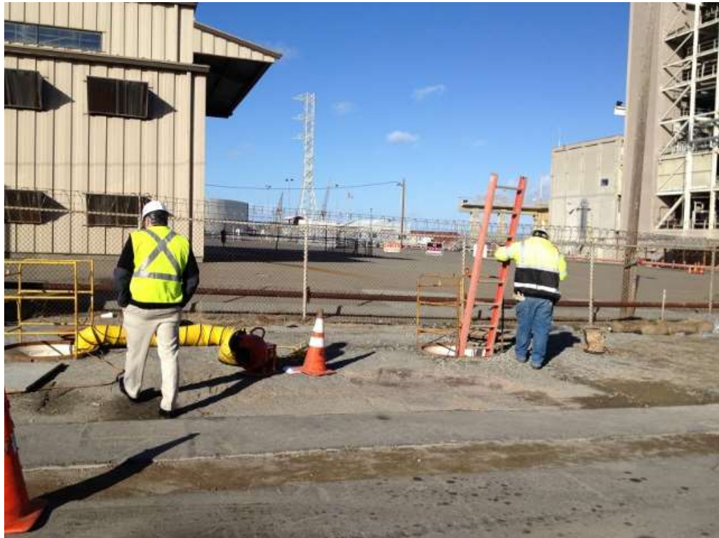
Figure 4 – Crew working in vault on 23 rd Street. View north, November 24, 2015.
