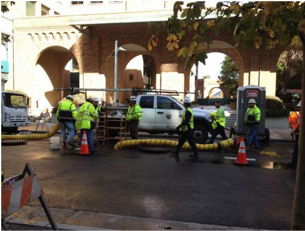
Figure 3 – Crew working in vault on Spear Street. View north, November 24, 2015.
