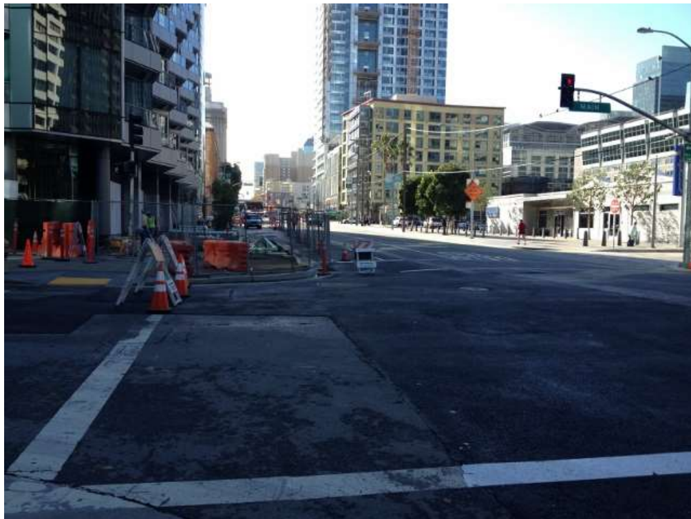
Figure 2 – Folsom Street repaved at Main Street. View south, November 24, 2015.
