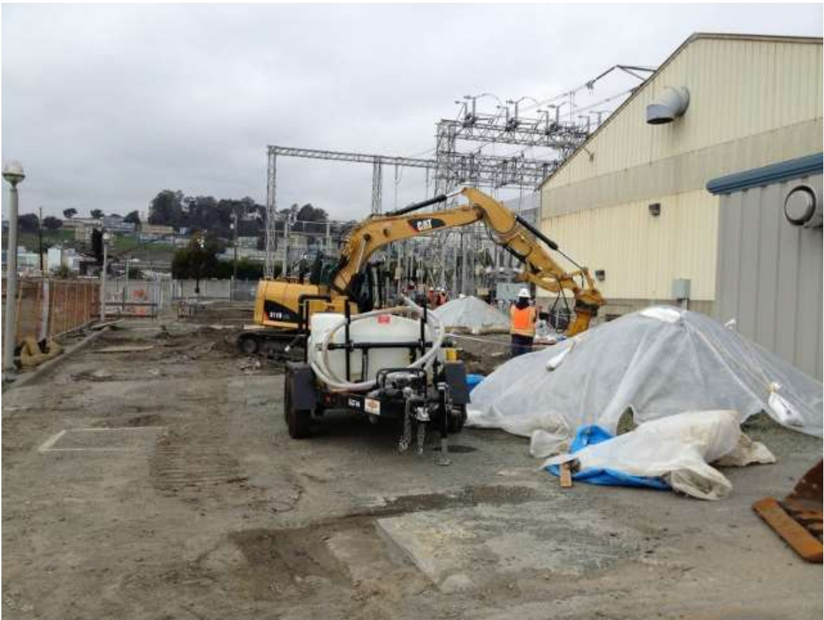
Figure 5 – Excavation work in substation adjacent to Potrero Switchyard. View west, December 17, 2015.
