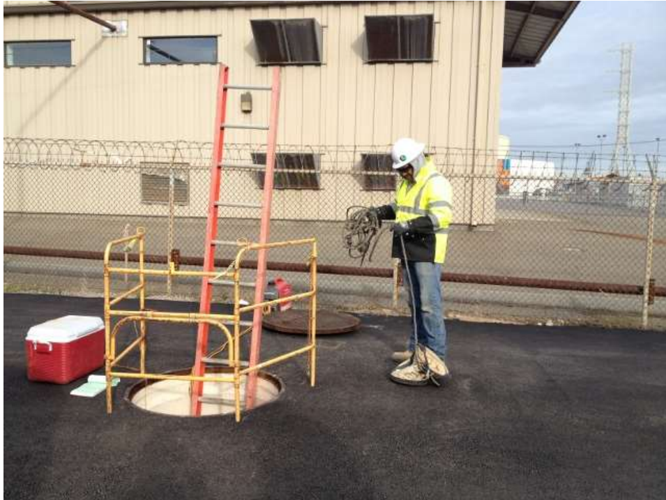
Figure 1 – Crew working in transition vault on 23 rd Street. View north, December 17, 2015.
