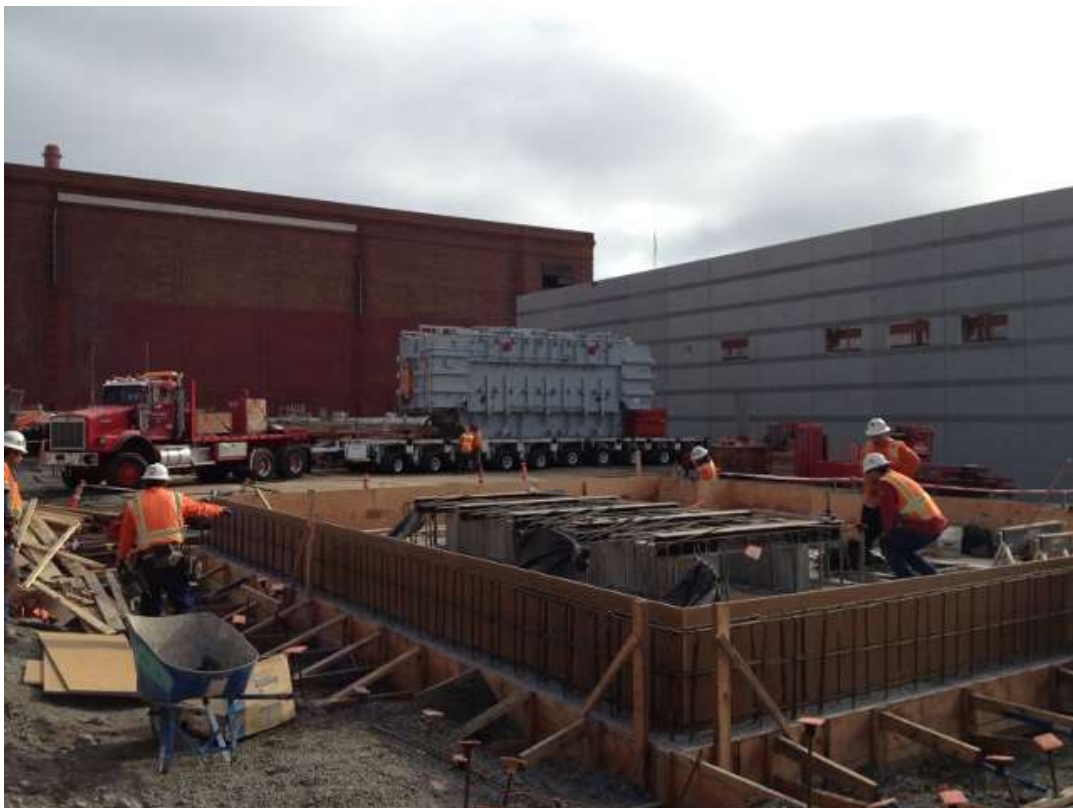
Figure 4 – Crews working on Reactor Pad in Potrero Switchyard. View southeast, December 17, 2015.
