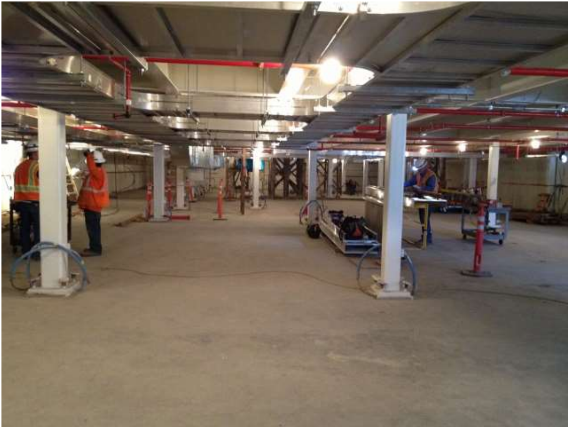
Figure 5 – Crews working inside the GIS building basement. View east, April 20, 2016.
