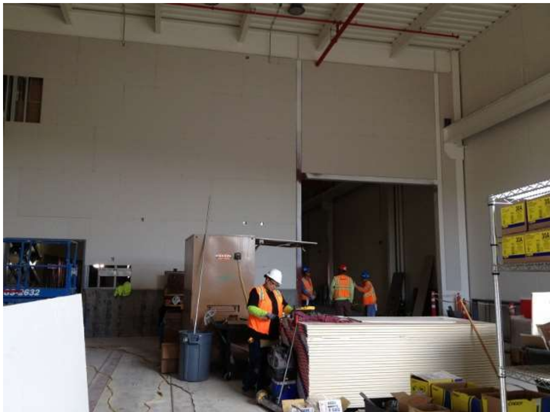
Figure 4 – Crews working inside the GIS building. View east, April 20, 2016.
