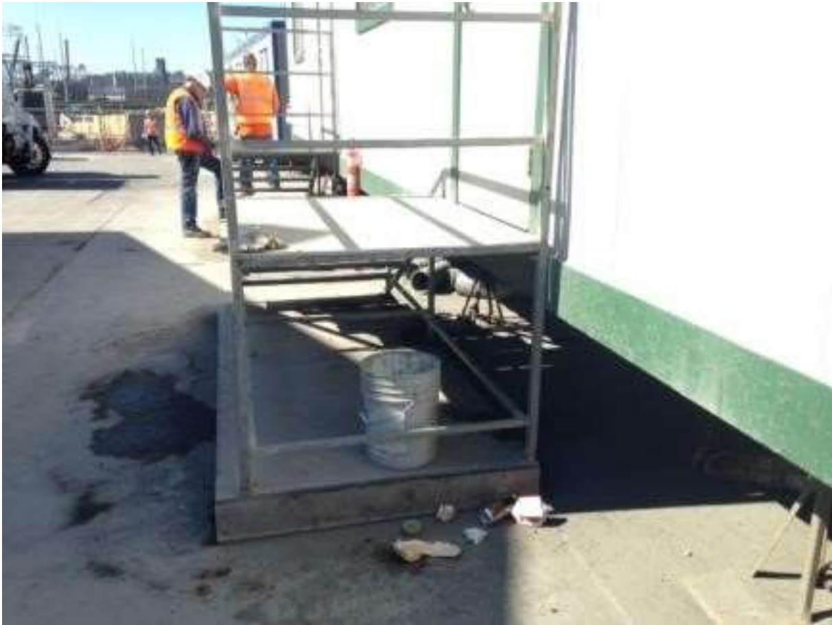
Figure 5: Litter accumulating around Potrero Switchyard, June 27, 2016. Photo courtesy of PG&E.
