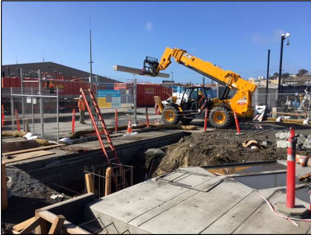
Figure 1 – Overaa offloading materials at Potrero Switchyard, October 17, 2016. Photo courtesy of PG&E.
