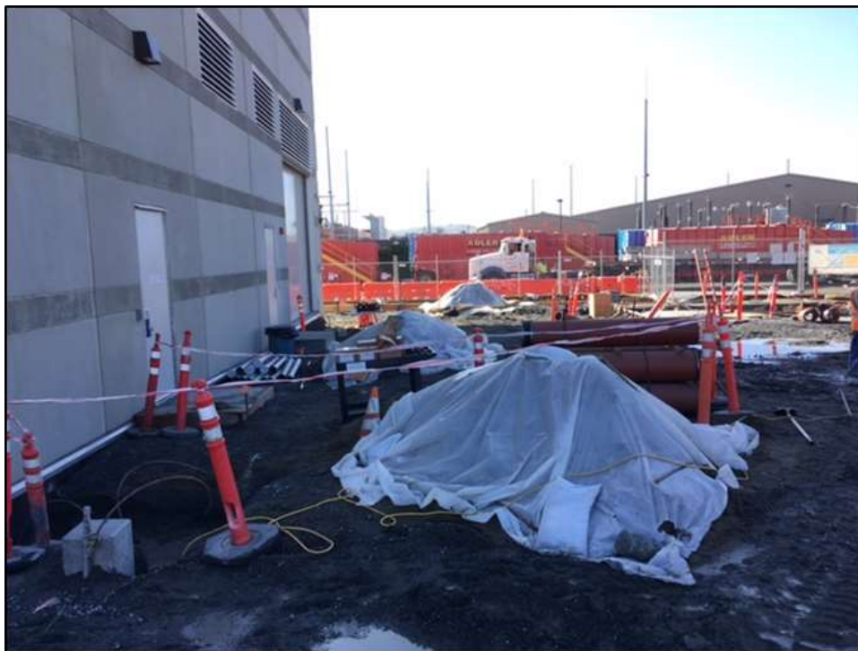
Figure 4 - SWPPP inspections at the Potrero Switchyard with stockpiles covered for rain event, October 17, 2016. Photo courtesy of PG&E.
