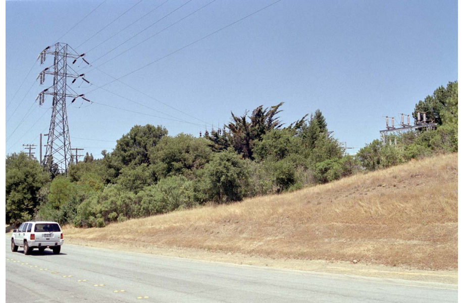
45. View of Carolands Substation from Skyline Boulevard looking northeast
