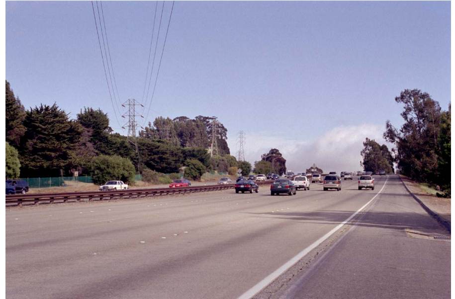
51. Transmission line crossing (near Milepost 9) north of Golf Course Blvd/ Hayne exit from southbound Interstate 280
