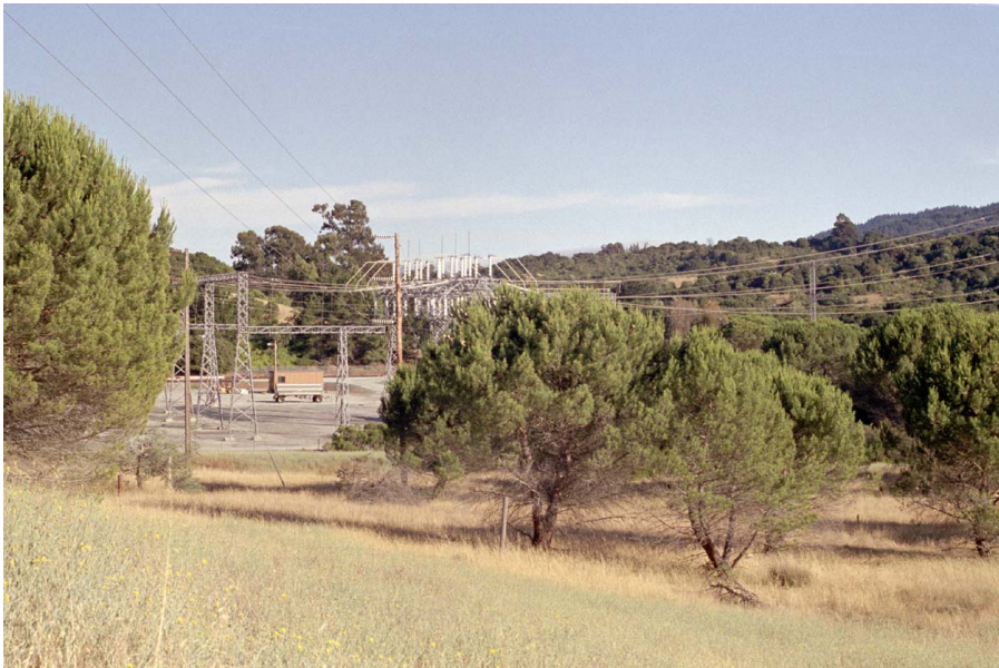
3. View of Jefferson Substation from Edgewood County Park looking south * Simulation view
