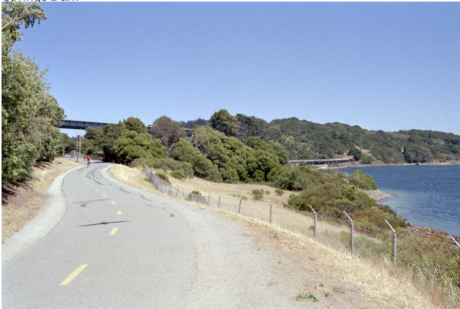
40. View of Crystal Springs Dam from the south end of Sawyer Camp Trail looking southeast
