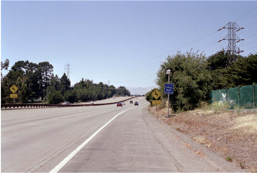
50. Transmission line crossing (near Milepost 9) north of Golf Course Blvd/ Hayne exit from northbound Interstate 280*
