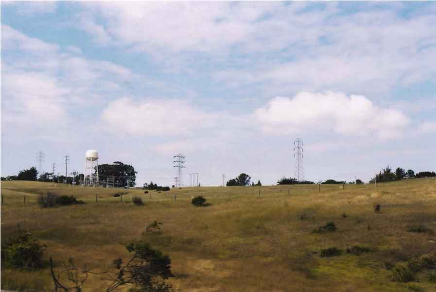
30. View from Highway 92 to Interstate 280 off-ramp looking northeast towards Ralston substation
