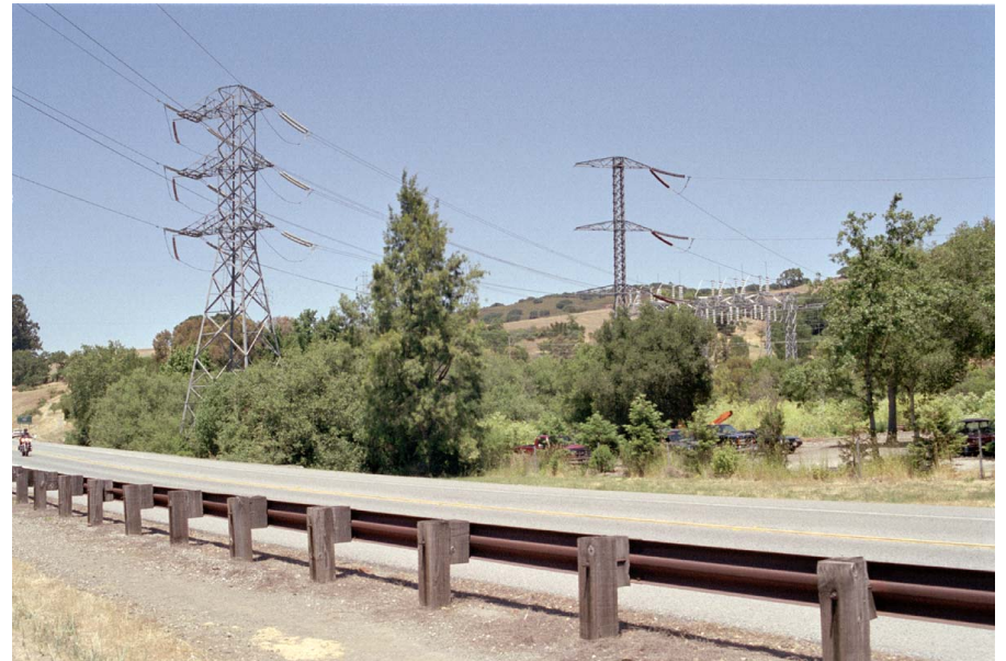
2. View of Jefferson Substation from Cañada Trail looking north*
