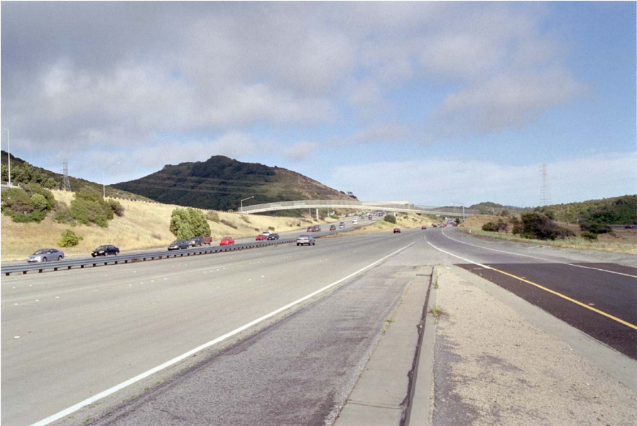
33. Transmission line crossing (near Milepost 5) south of Highway 92 from southbound Interstate 280*
