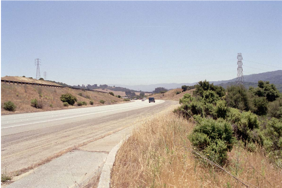
32. Transmission line crossing (near Milepost 1.5) north of Jefferson Substation from southbound Interstate 280*
