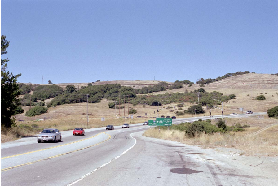
29. View from Highway 92 near Reservoir looking east
