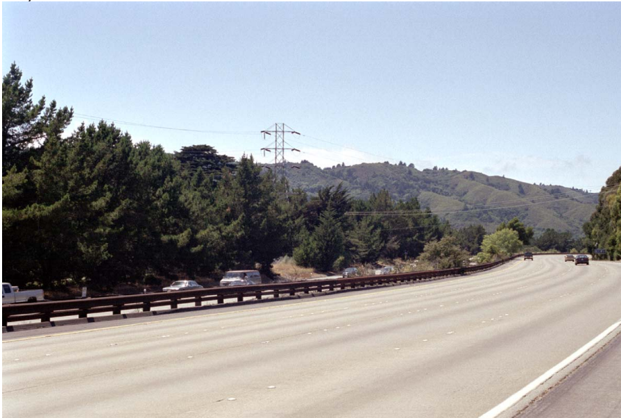
52. Transmission line crossing (near Milepost 10.5) at Summit Drive from northbound Interstate 280
