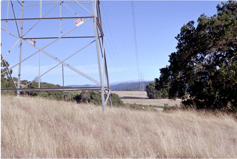
6. View from Edgewood County Park looking south
