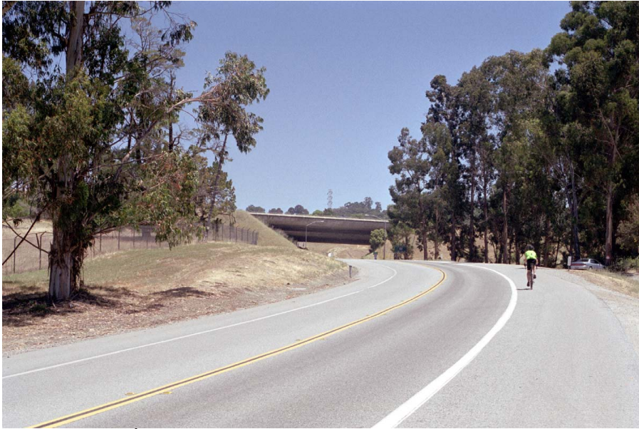
9. View from CaOada Road looking southwest toward Interstate 280 underpass
