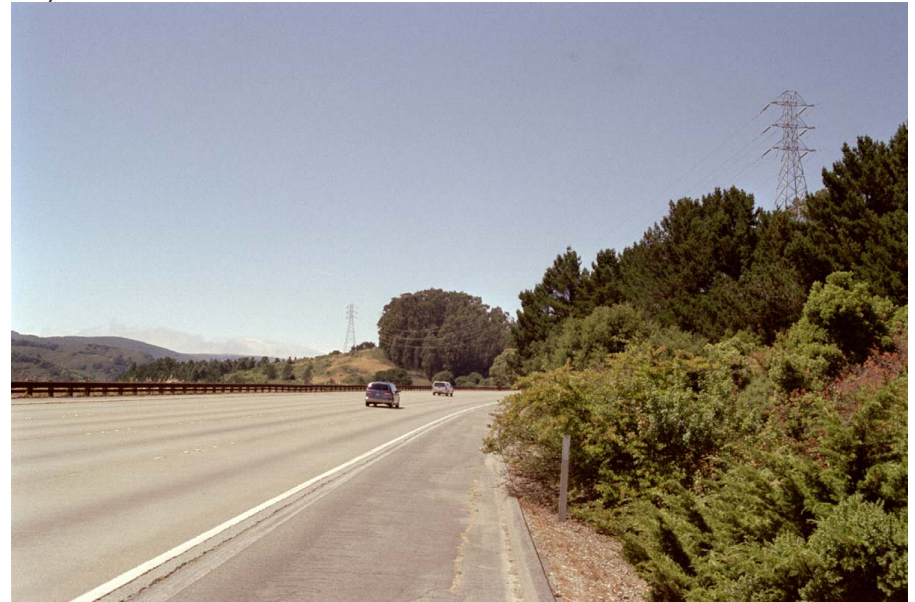
53. Transmission line crossing (near Milepost 11) at Skyline Park from northbound Interstate 280
