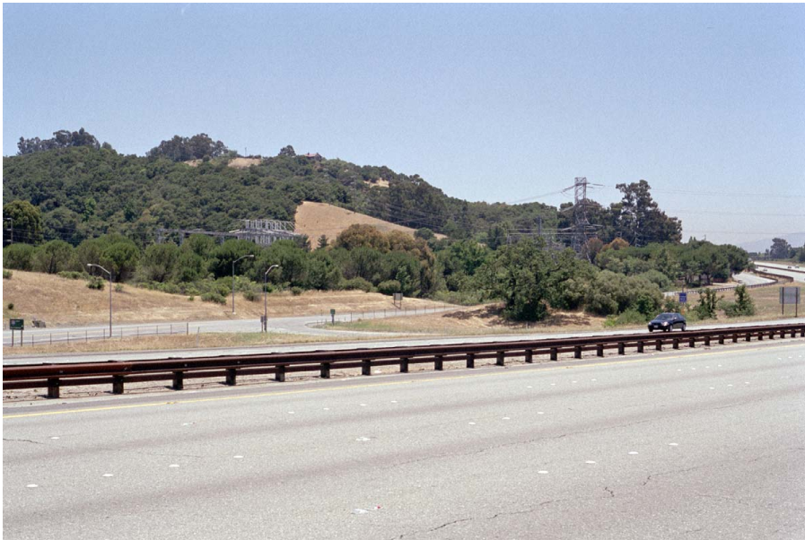
1. View of Jefferson Substation from southbound Interstate 280
