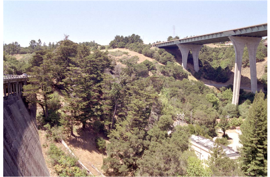
39. View of Crystal Springs Substation and Dam from northbound Skyline Boulevard
