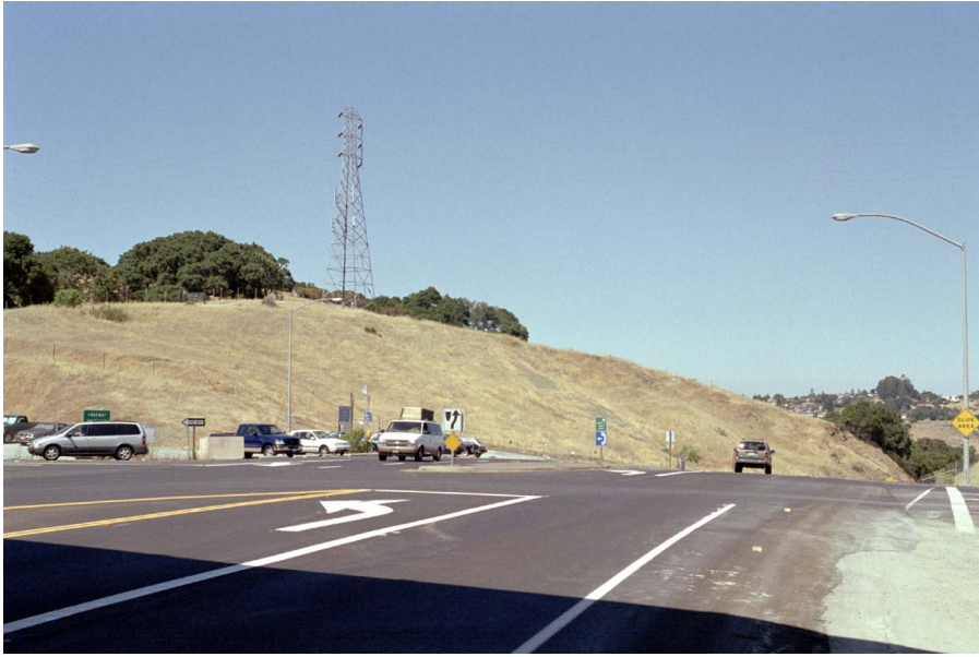
10. View from Edgewood Road at Interstate 280 looking east
