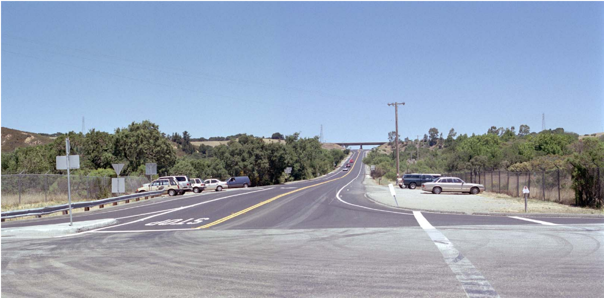
11. View from CaOada Road looking east along Edgewood Road toward Interstate 280
