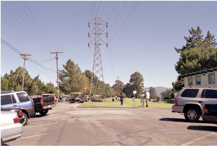
55. View of Crystal Springs Golf Course parking lot and putting greens looking southeast
