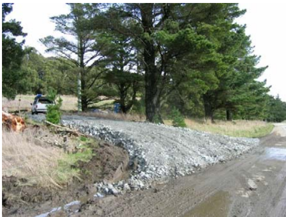
Figure 2-9. Access road to Tower #86, re-rocked (Segment 2 overhead, 2-2-06)
