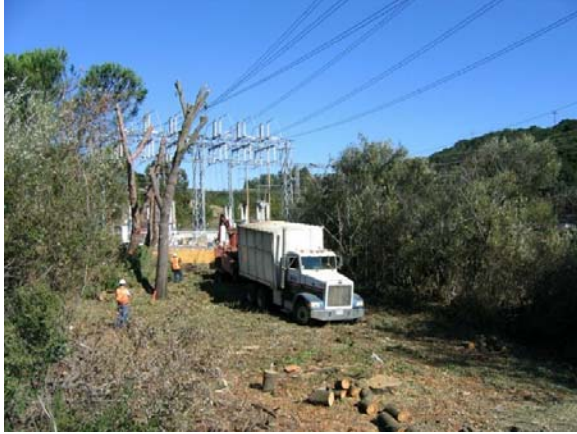
Figure 3-3. Tree removal for trench alignment into Jefferson Substation (10-25-05)
