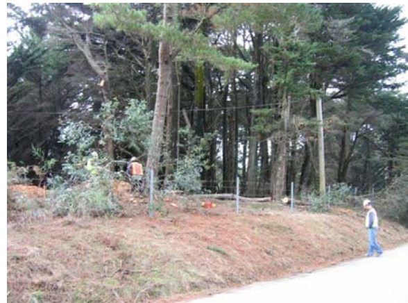
Figure 2-8. Tree trimming between Pole #74 and Hillcrest (Segment 2 overhead, 11-29-05)
