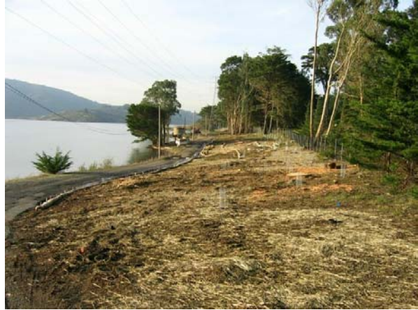
Figure 2-15. Restoration between Towers #83 and #84 (Segment 2 overhead, 1-5-06)
