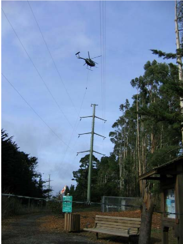
Figure 2-12. Helicopter starting to fly sock line from Tower #77 (Segment 2 overhead, 1-11-06)
