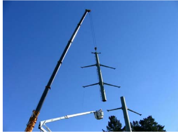
Figure 2-11. Setting top of Tower #82A (Segment 2 overhead, 2-07-06)
