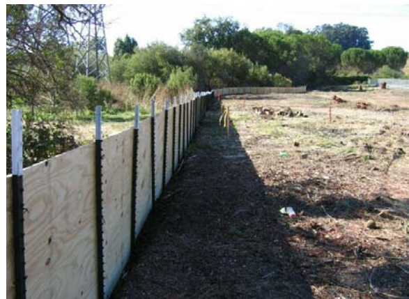
Figure 3-2. Jefferson Substation, plywood fence installation around expansion area (9-15-05)
