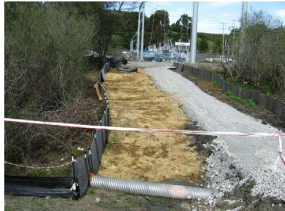
Figure 3-4. Updated erosion controls on right-of-way into Jefferson Substation (4-13-06)
