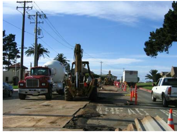
Figure 2-20. Trenching activities very dirty on Hillside (Segment 4, 10-27-05)
