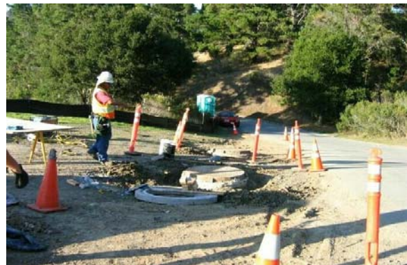
Figure 2-6. San Francisco Public Utilities Commission watershed, Manhole #38 (Segment 2 underground, 11-16-05)
