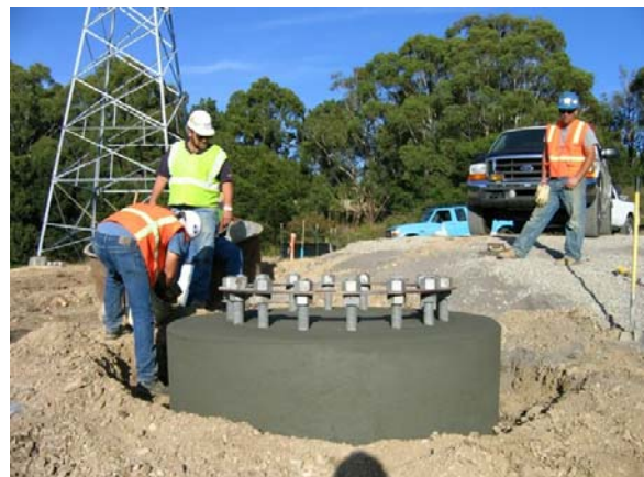
Figure 2-7. Foundation #70A (Segment 2 overhead, 10-17-05)
