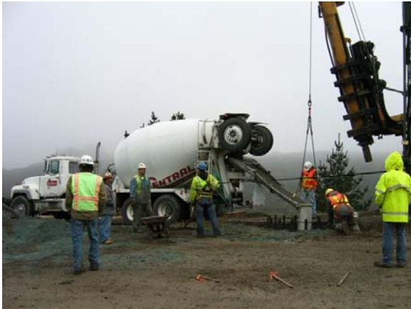
Figure 2-10. Pouring slurry for Foundation #93 (Segment 2 overhead, 11-29-05)
