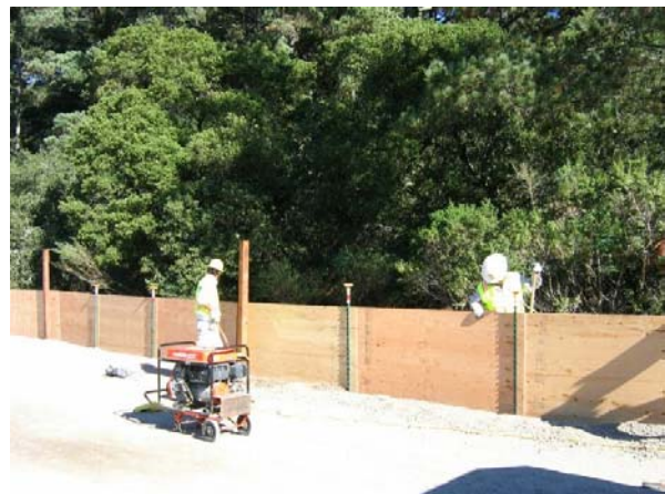
Figure 2-14. Crews building fence around staging yard (Segment 2 overhead, 10-5-05)
