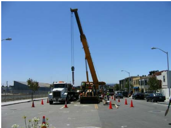
Figure 2-16. Setting Manhole #46 on Huntington Drive (Segment 3, 7-1-05)
