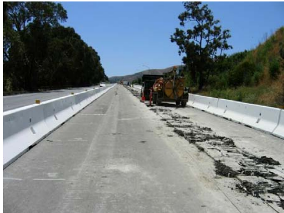
Figure 2-22. Trenching area along Bayshore blocked off by k-rail (Segment 5, 6-4-05)
