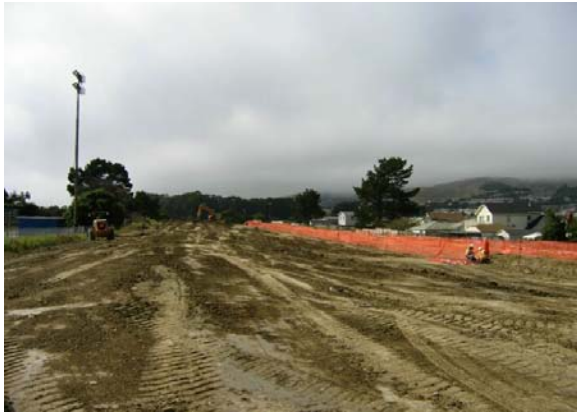
Figure 2-19. BART right-of-way north of South Spruce Street (Segment 4, 7-6-05)
