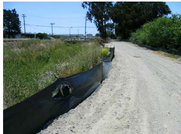
Figure 2-17. Silt fence around wetland (Segment 4, 6-24-05)
