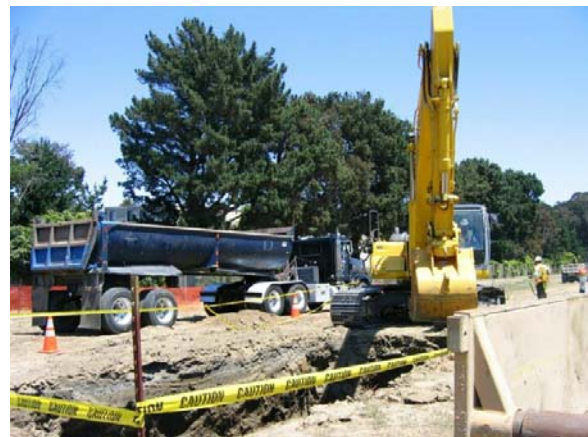
Figure 2-18. Bore pit excavation in BART right-of-way (Segment 4, 7-15-05)
