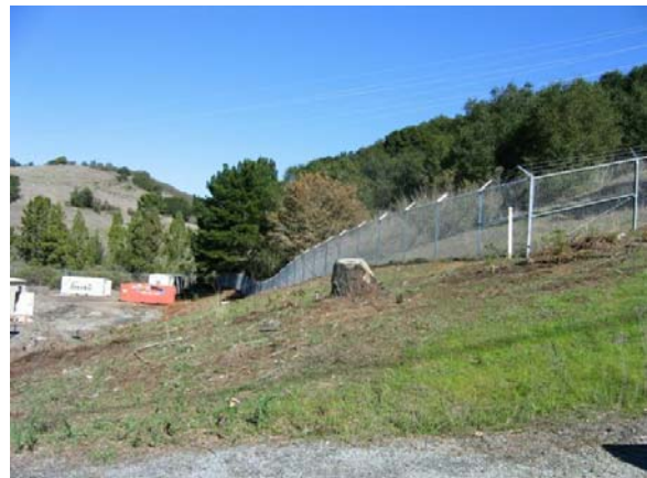
Figure 3-1. New fence at Jefferson Substation on eastern side (2-07-06)
