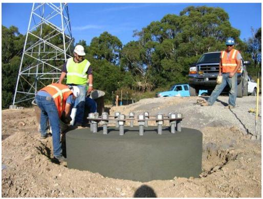
**Figure 2** – Foundation for Pole #70A in SFPUC Watershed, Segment 2 Overhead, October 17, 2005.
