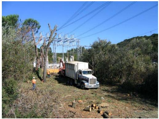
**Figure 7** – Tree and brush clearing for the trench alignment into the Jefferson Substation from Manhole #1, October 25, 2005.
