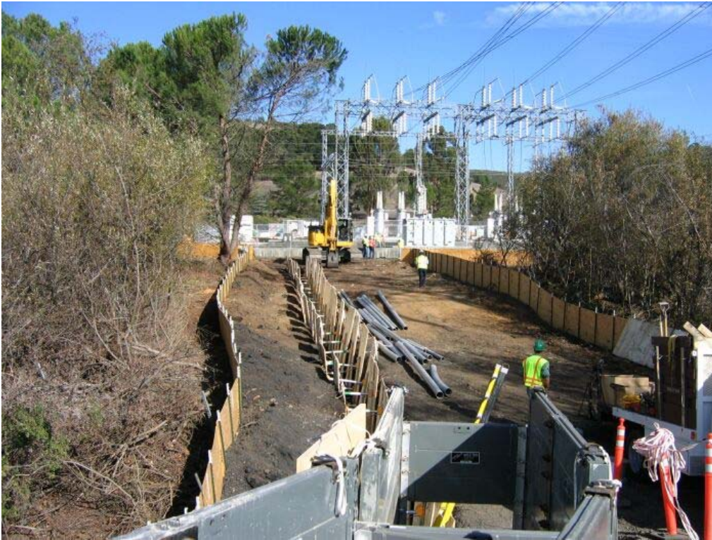
Figure 6 – Trench into Jefferson Substation from Manhole #1, November 18, 2005
