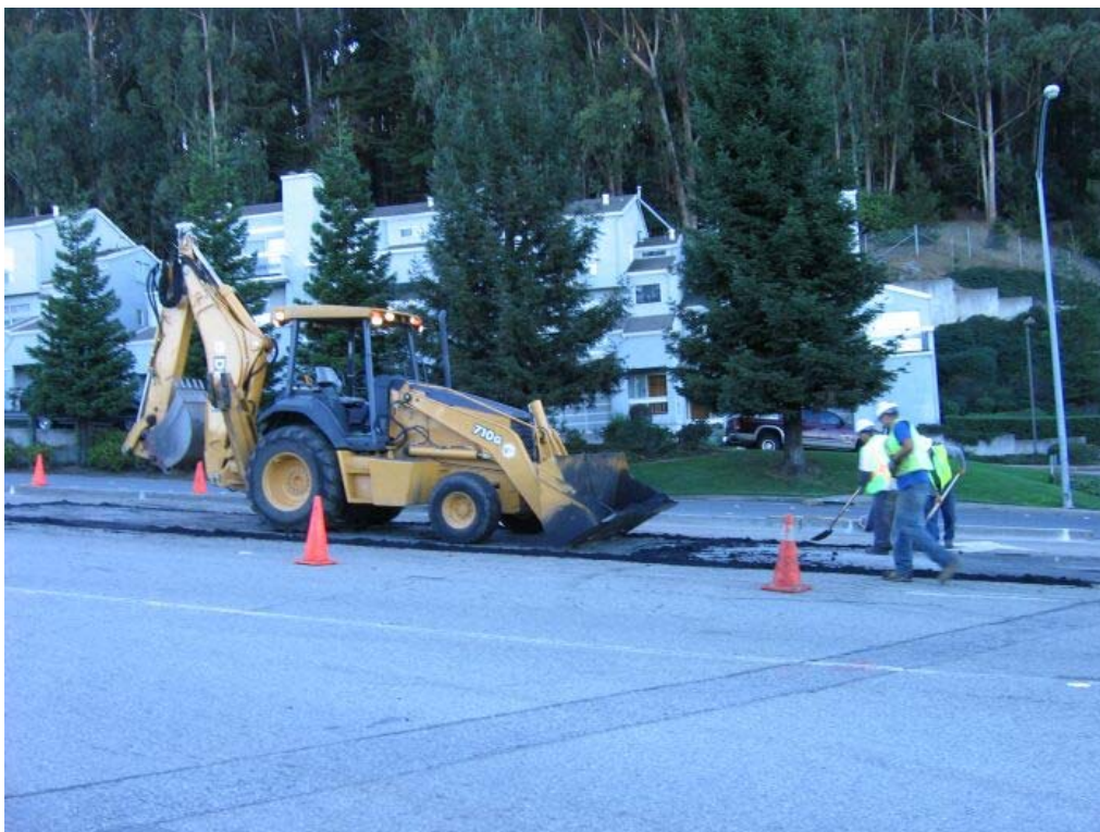
Figure 4 – Crews conducting trenching activities on San Bruno Avenue, Segment 3, November 15, 2005.
