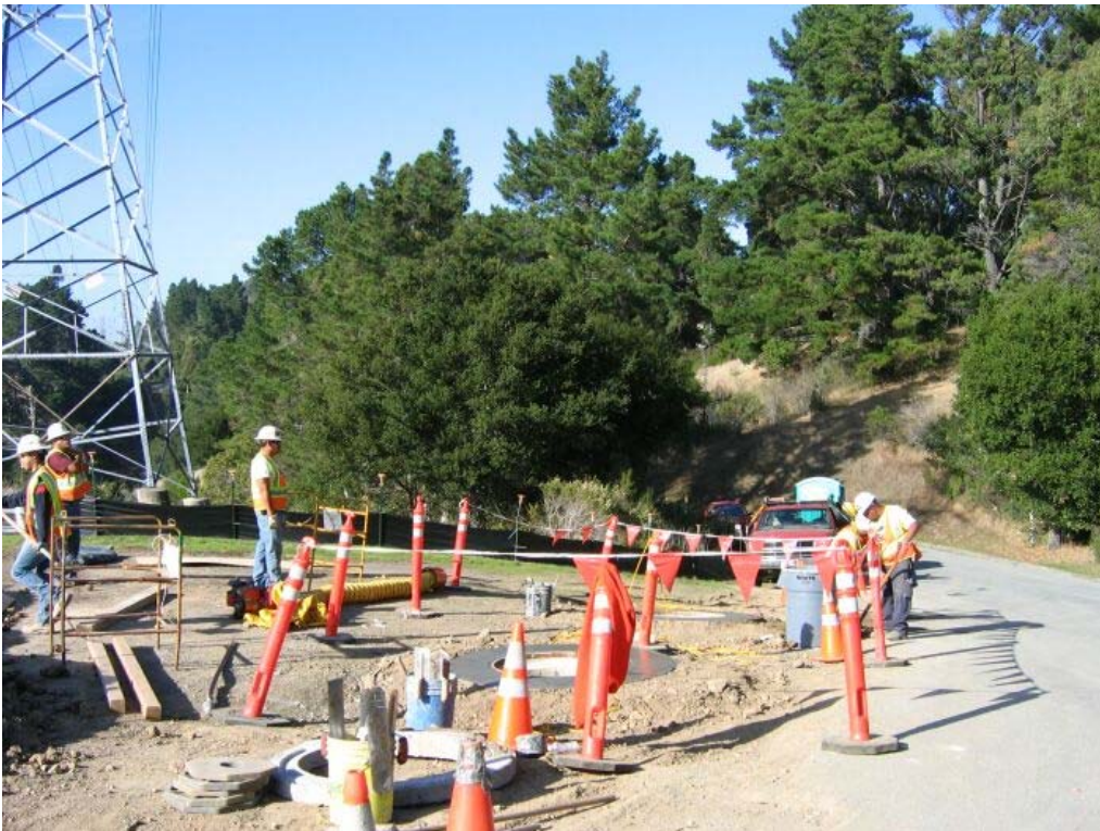
Figure 2 – Crews working in SFPUC Watershed on Manhole #38, Segment 2 Underground, November 18, 2005.
