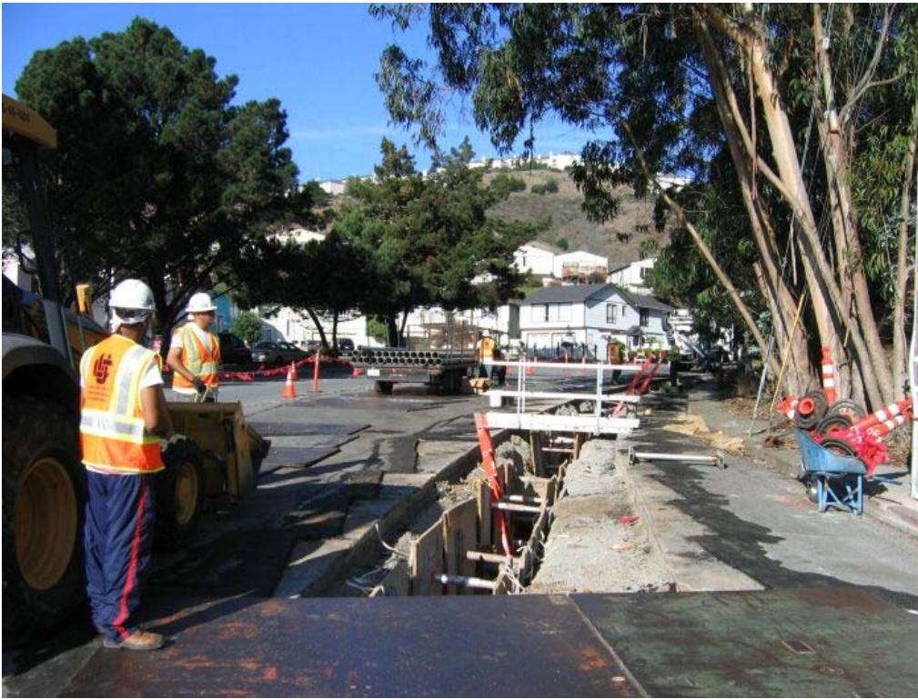
Figure 5 – Trenching activities on East Market in Daly City, Segment 5, November 21, 2005
