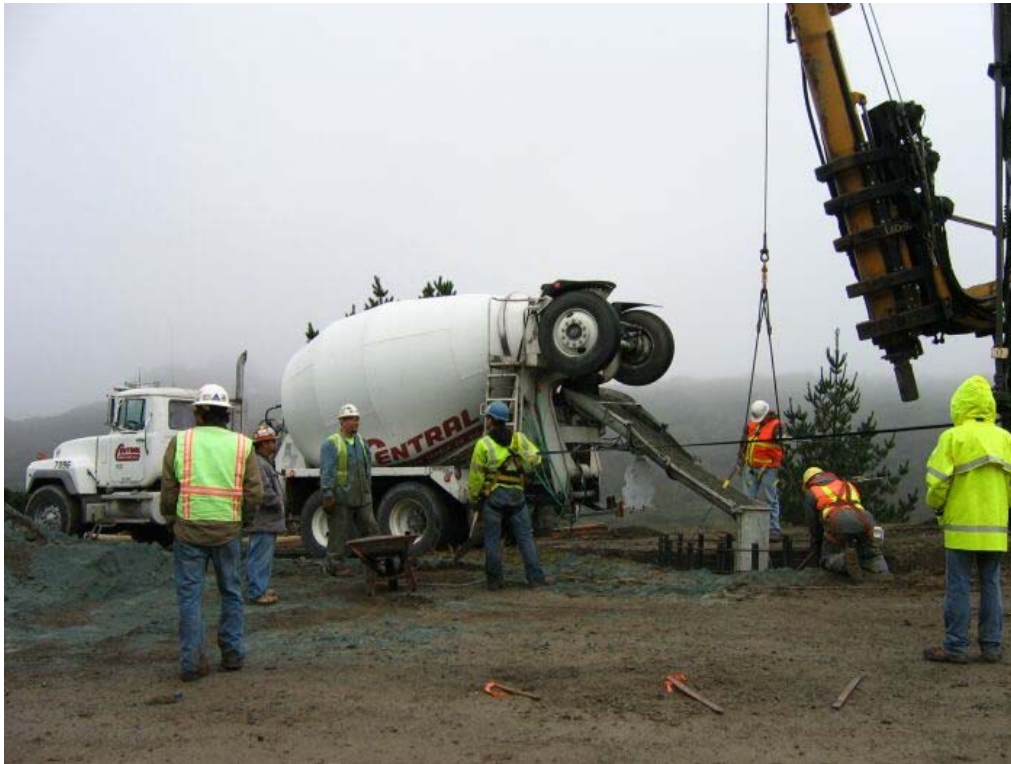
Figure 3 – Crews pouring cement for foundation for Tower #93, Segment 2 Overhead, November 29, 2005
