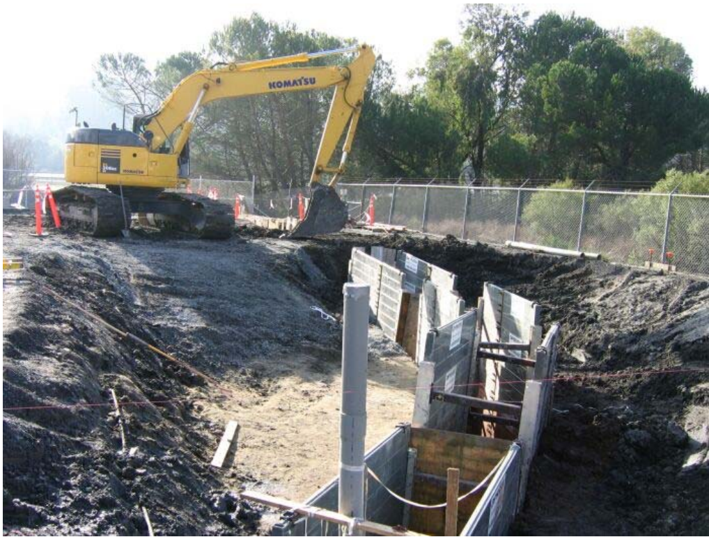
Figure 5 – Trenching activities into the Jefferson Substation, January 10, 2006.
