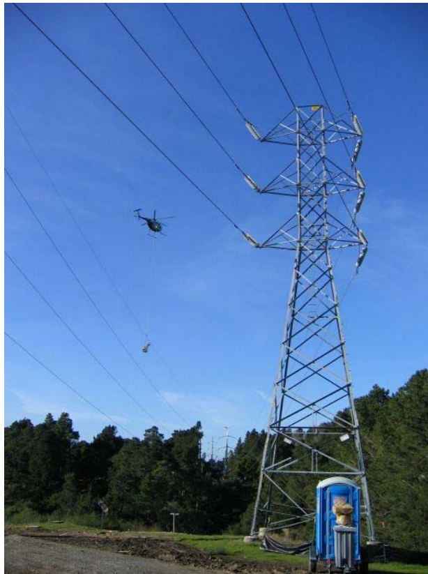
Figure 3 – Helicopter dangling a man in a basket who is attaching bird diverters to the OPGW line between Towers #70A and #71, Segment 2 Overhead, January 19, 2006.
