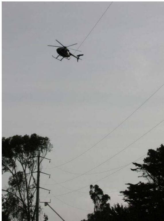
Figure 2 – Helicopter flying sock line toward Tower #76 from Tower #77, Segment 2 Overhead, January 11, 2006.
