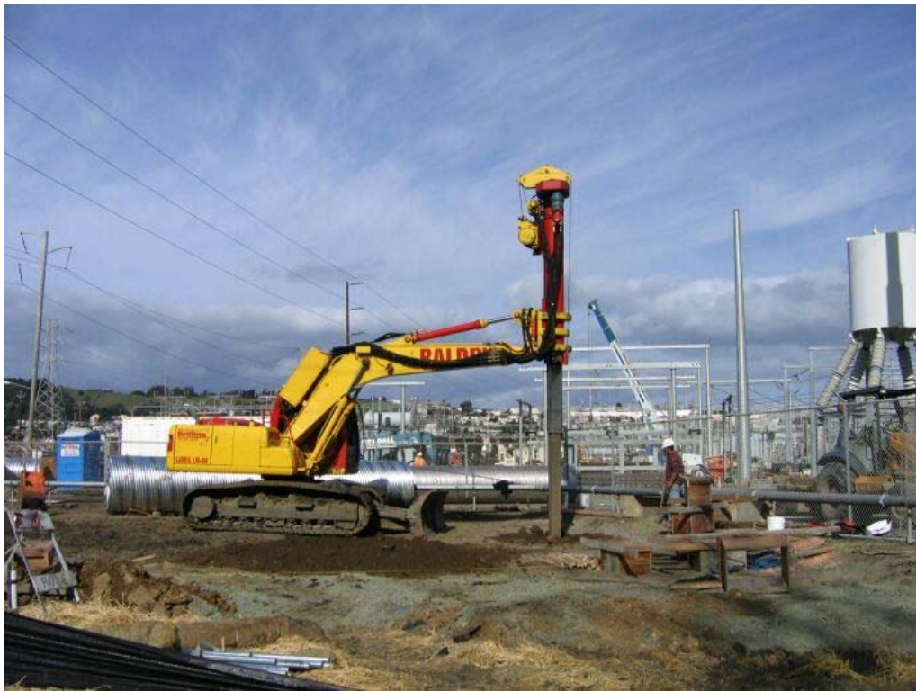
Figure 6 – Drilling tower foundation pits at the Martin Substation, January 25, 2006.
