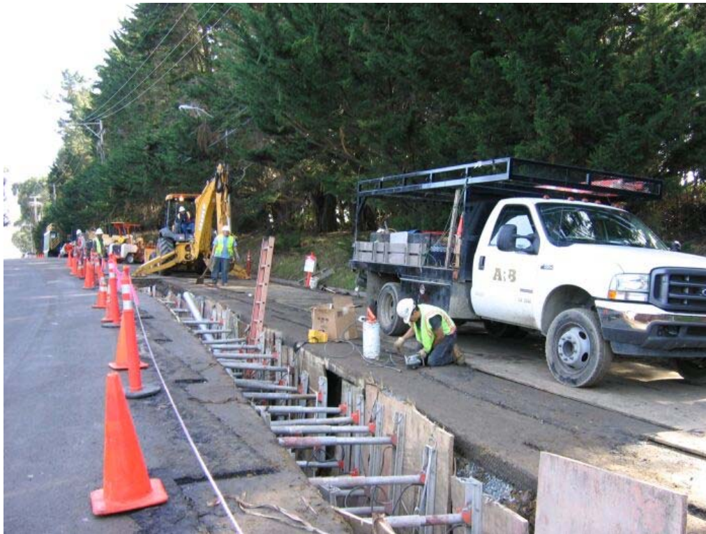
Figure 4 – Trenching activities on Glenview Drive, Segment 3, January 18, 2006.
