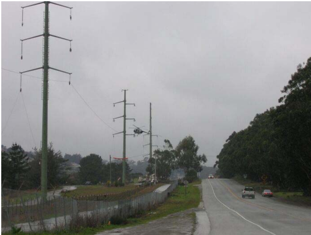
Figure 4 – Helicopter flying sock line from Tower #82 through Tower #93, Segment 2 Overhead, February 17, 2006.
