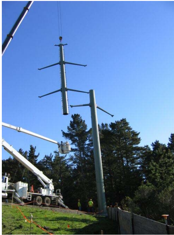
Figure 3 – Crews setting top portion of Tower #82A, Segment 2 Overhead, February 7, 2006.
