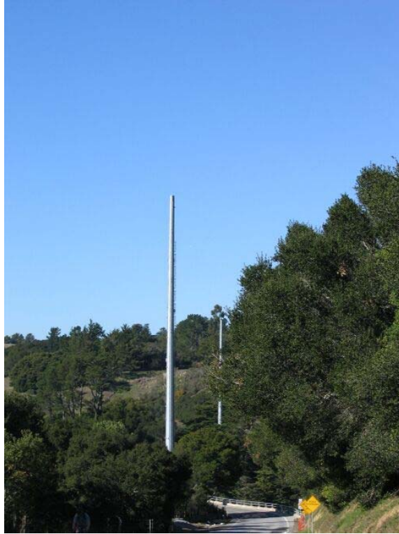
Figure 1 – View looking north at towers on either side of Crystal Springs Dam, Segment 1, February 7, 2006.
