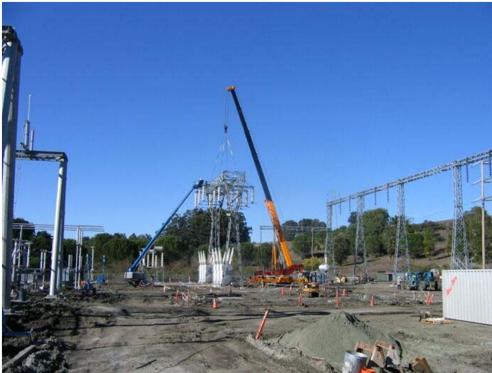
Figure 6 – Crews working with crane from lift at the Jefferson Substation, February 7, 2006.
