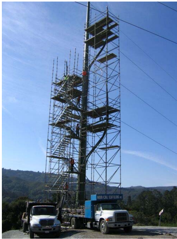
Figure 5 – Scaffolding built around Tower #70A, Segment 2 Overhead, February 24, 2006.
