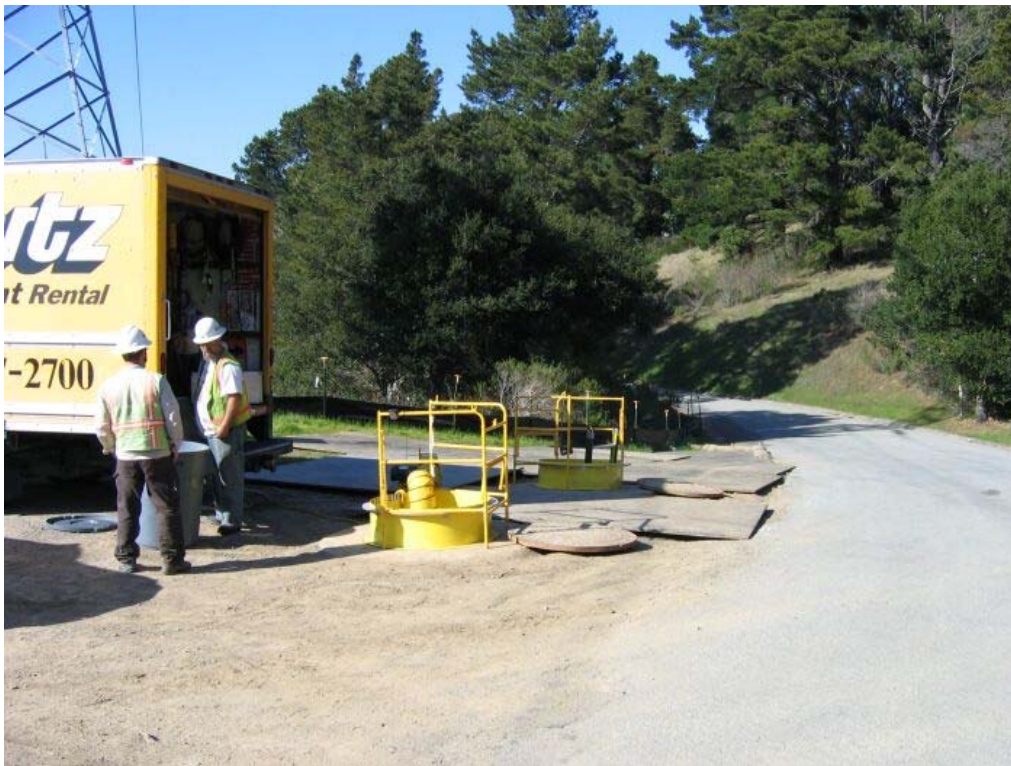
Figure 2 – Crews splicing at Manhole #38, Segment 2 Underground in the SFPUC watershed, February 24, 2006.
