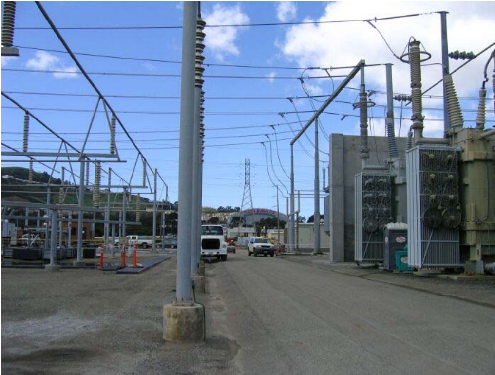
Figure 5 – New construction at the substation, Martin Substation, April 17, 2006.
