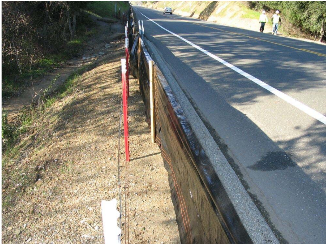
Figure 1 Exclusion Fencing along west side of Canada Road just north of the Pulgas Water Temple January 20, 2005
