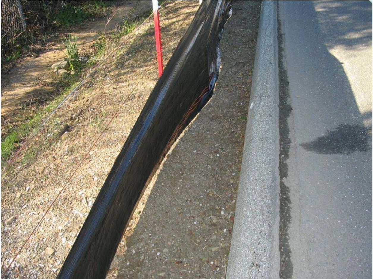
Figure 2 Exclusion Fencing along west side of Canada Road just north of the Pulgas Water Temple January 20, 2005
