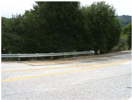
**Figure 3** – Trench plated recessed into pavement in Caltrans ROW on Skyline, Segment 1, February 23, 2005
