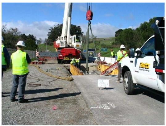
**Figure 1** – Manhole #1 setting vault in pit with crane on Cañada Road, Segment 1, February 23, 2005
