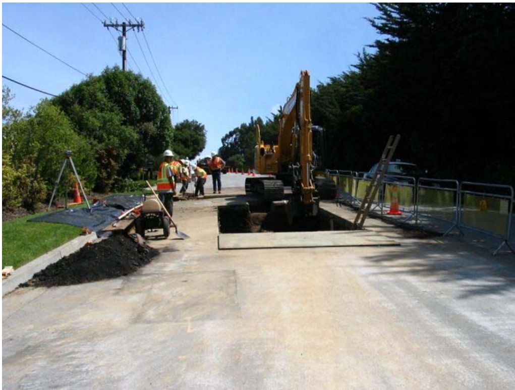
Figure 3 – Crews excavating Manhole #34 on Skyline Boulevard, Segment 2, April 29, 2005.
