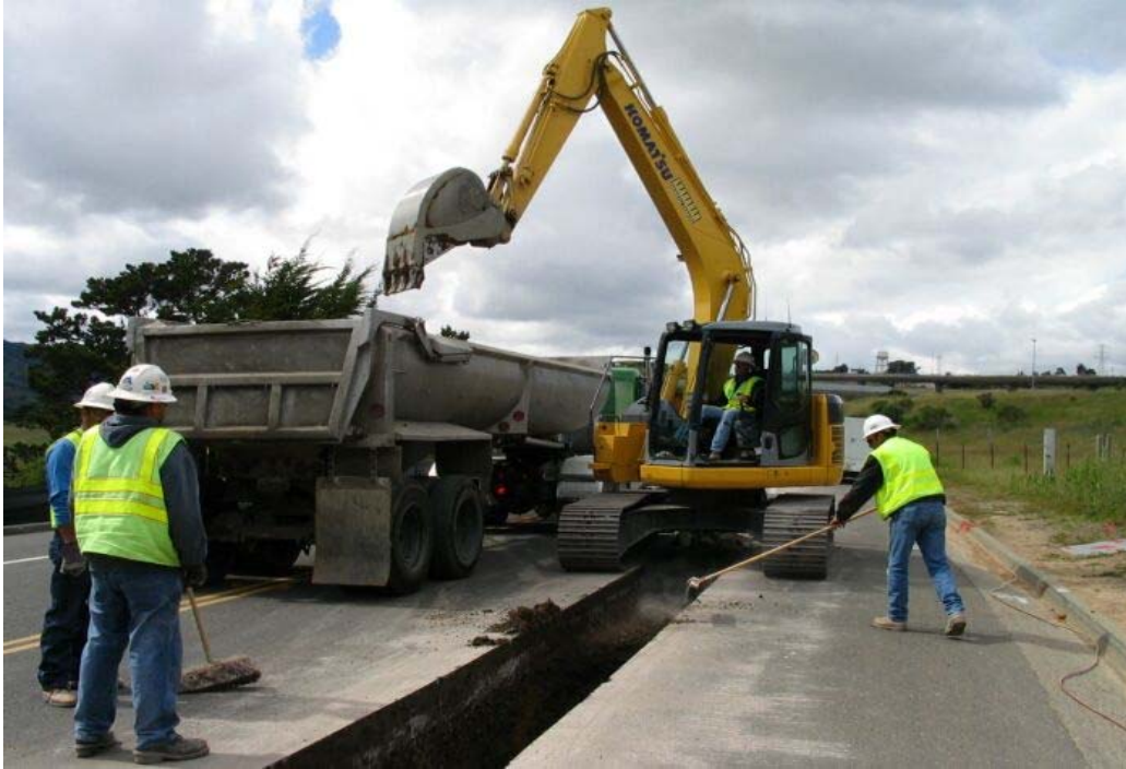
Figure 1 – Crews excavating trench north of Manhole #14 on Cañada Road, Segment 1, April 27, 2005.
