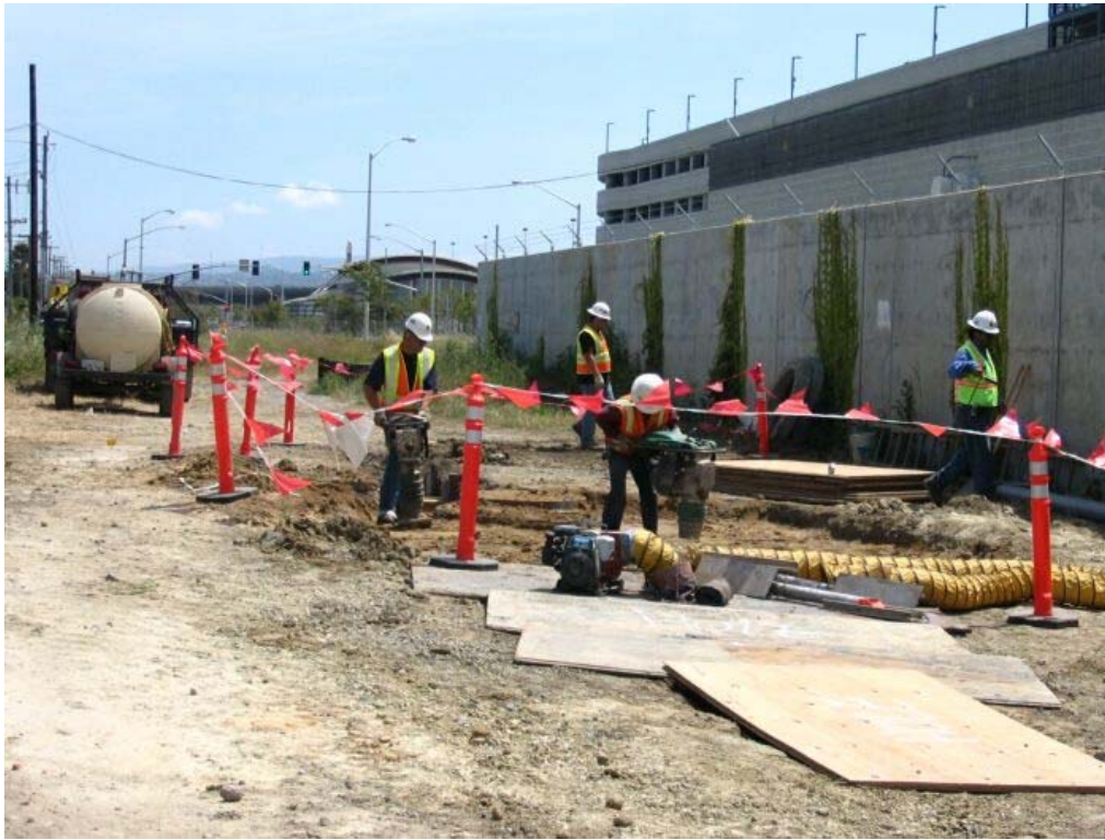
Figure 3 – Crews compacting soil over Manhole #48 in the BART right-of-way, Segment 4, May 12, 2005
