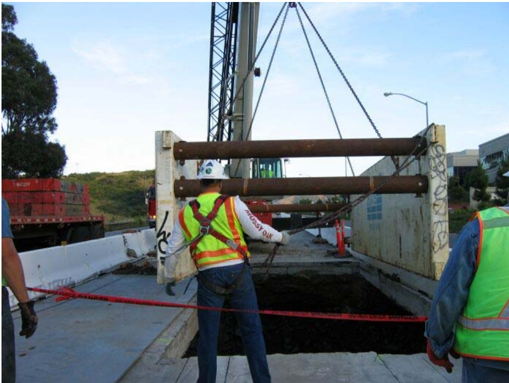
Figure 4 – Shoring being installed at Manhole #77 on Bayshore Boulevard, Segment 5, June 3, 2005
