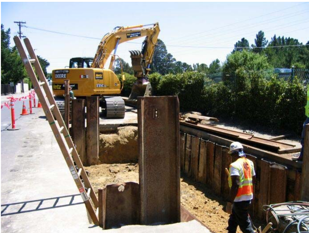
Figure 2 – Crews shoring Manhole #30 on Skyline Boulevard, Segment 2 Underground, June 1, 2005
