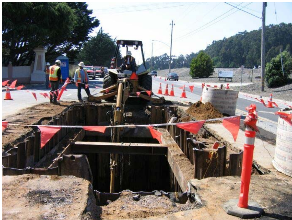
Figure 4 – Crews working at Manhole #59 on Hillside Drive, Segment 4, July 14, 2005
