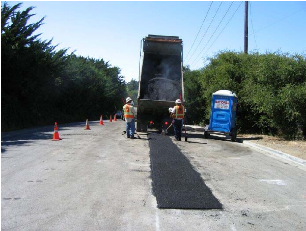
Figure 2 – Crews paving on Skyline Boulevard between Manholes #34 and #35, Segment 2 Underground, July 15, 2005
