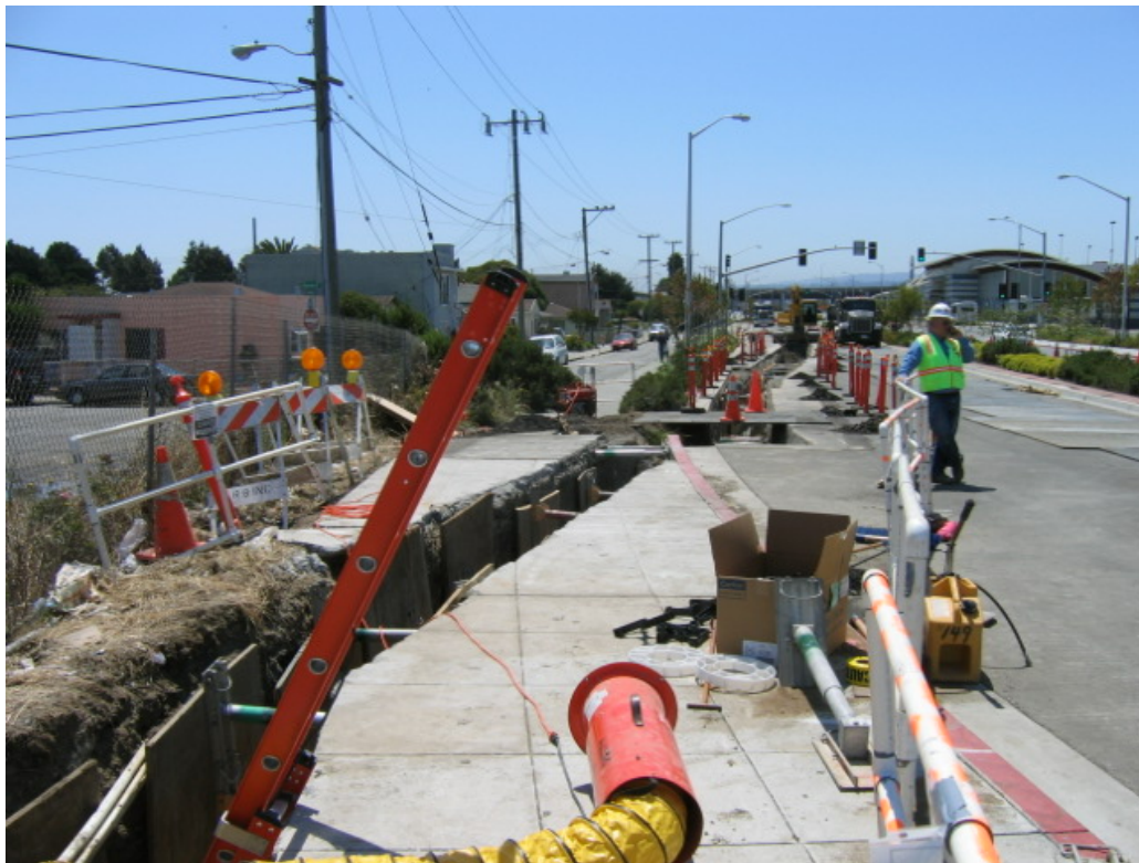
Figure 3 – Trenching operation along Huntington Ave, Segment 3, July 14, 2005.
