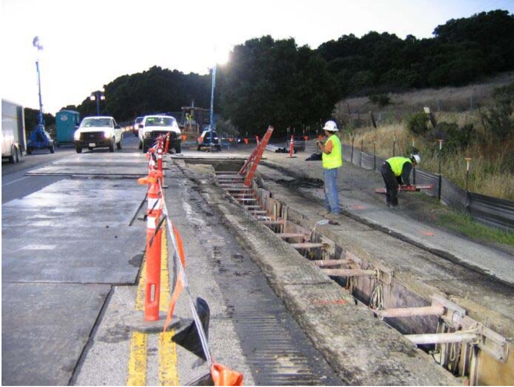
Figure 1 – Night trench work between Manholes #19 and #18, Segment 1, July 13, 2005
